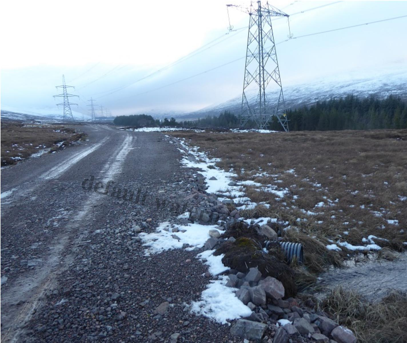
No work has been undertaken to narrow the track from 5m in width and no work undertaken to conceal plastic culvert
