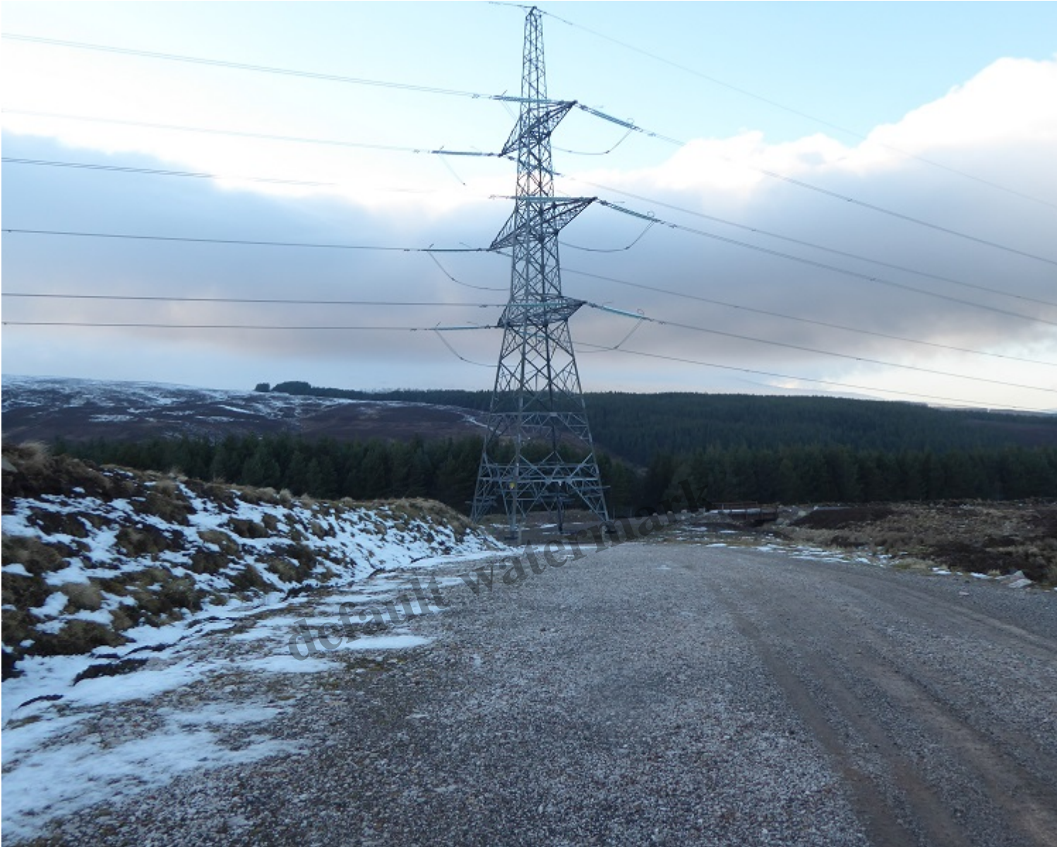
Another view of one side of the hammerhead. All this ground should have been restored.
