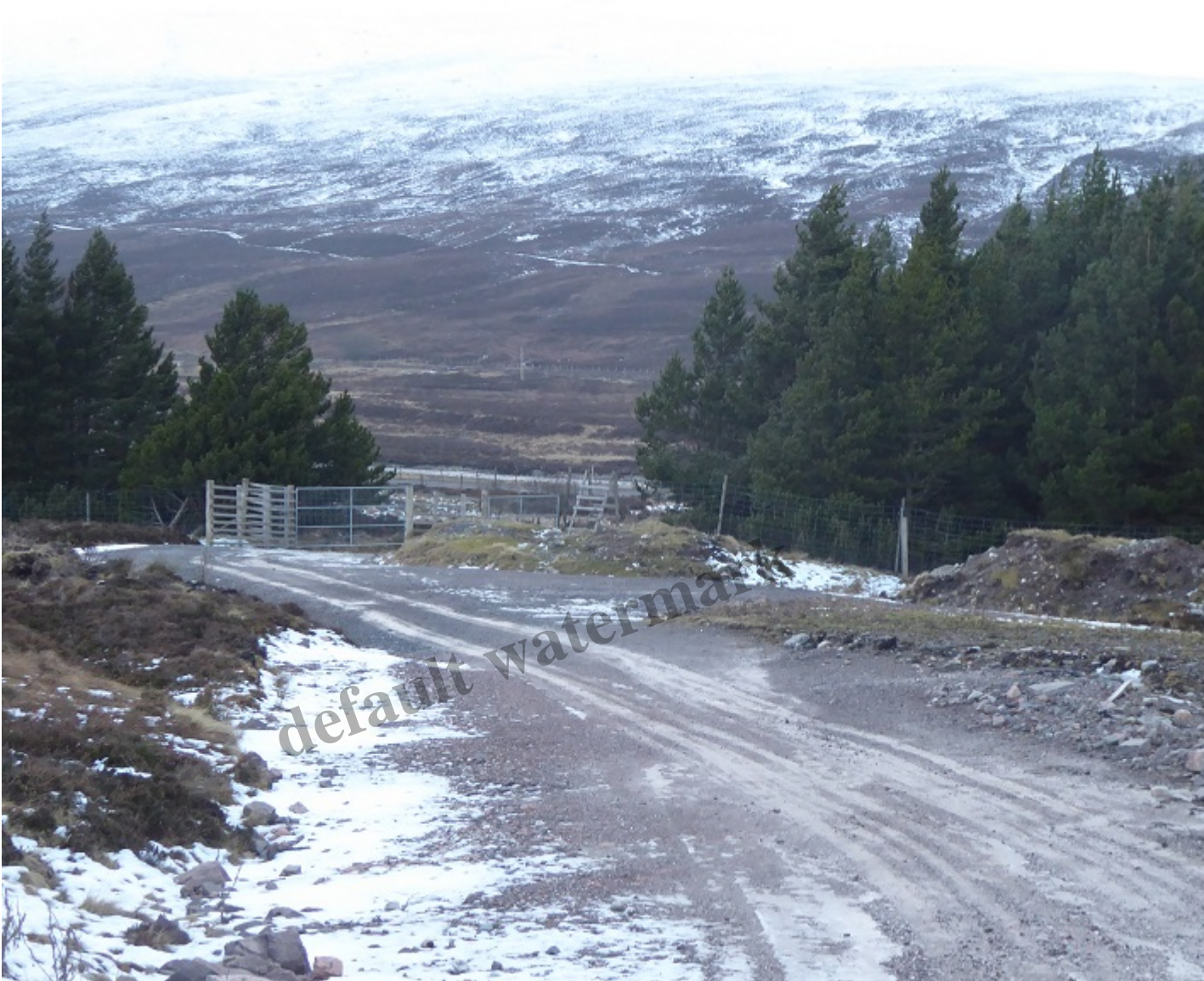
The access to the A9, more spoil heaps on right. The shelter belt helps conceal this mess.
