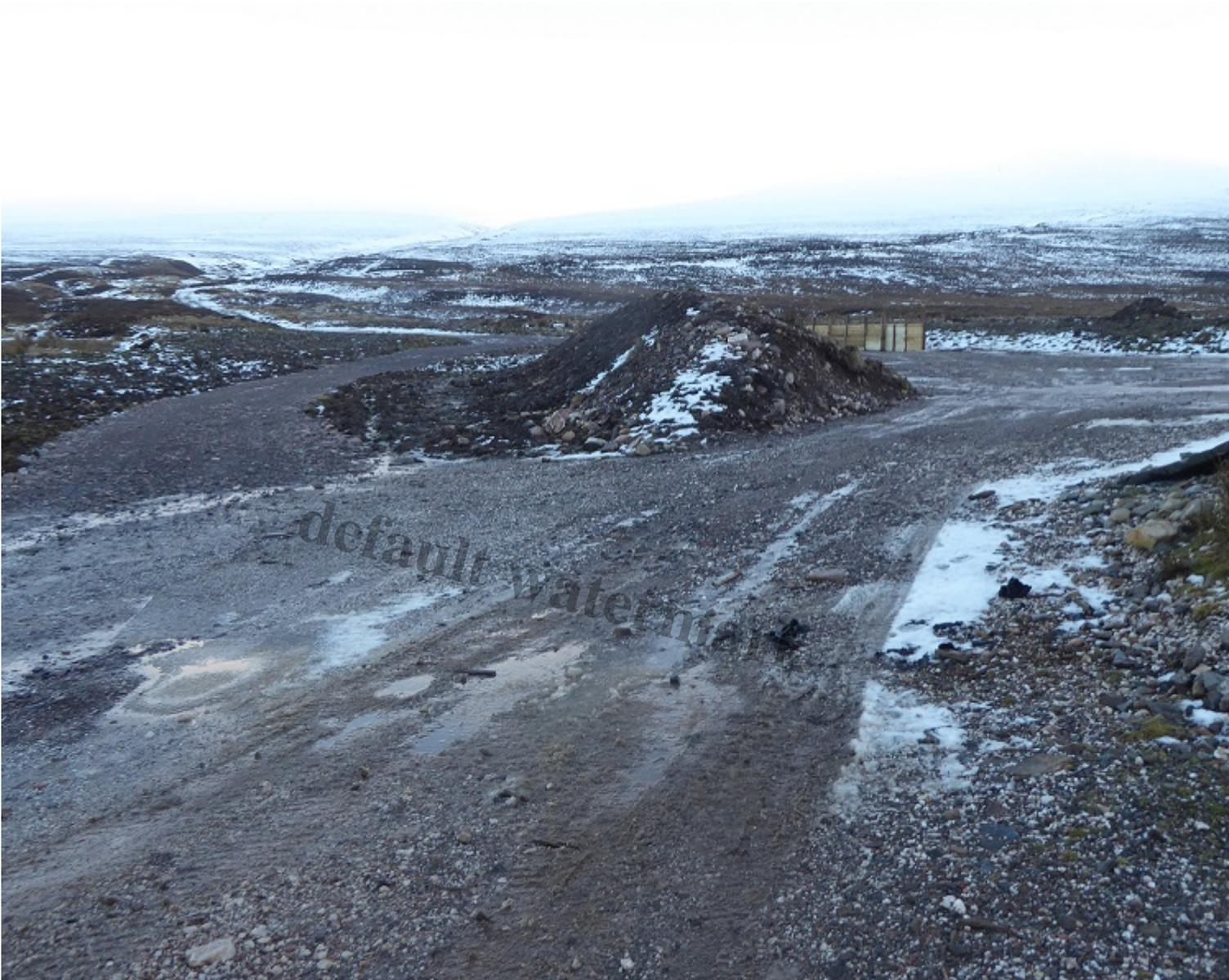
Part of the restoration proposed by the estate was removal of this hammerhead. Nothing has been done. There are piles of spoil in the centre and along right side of the area.
