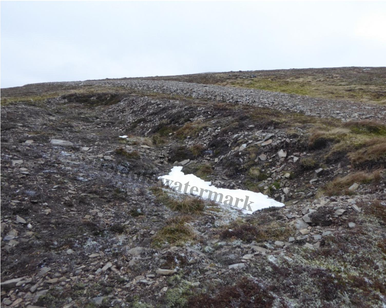
The aggregate has been 'won' from borrow pits at the side of the track, adding to the destruction of the summit heath.
