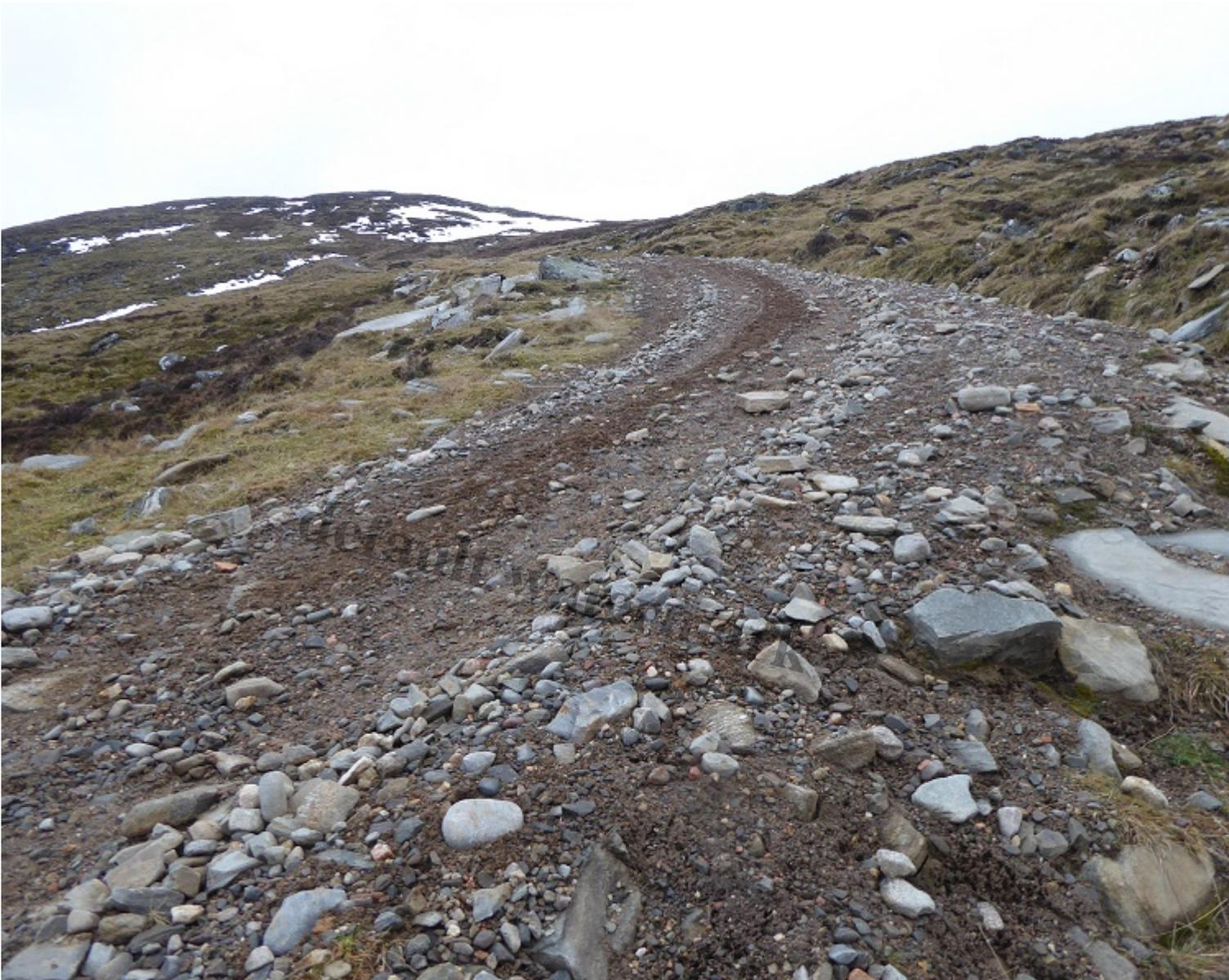
The older section of the track is too steep – far steeper than in SNH’s Guidance on Hill tracks – and is eroding. Its only a matter of time before this track washes out.
