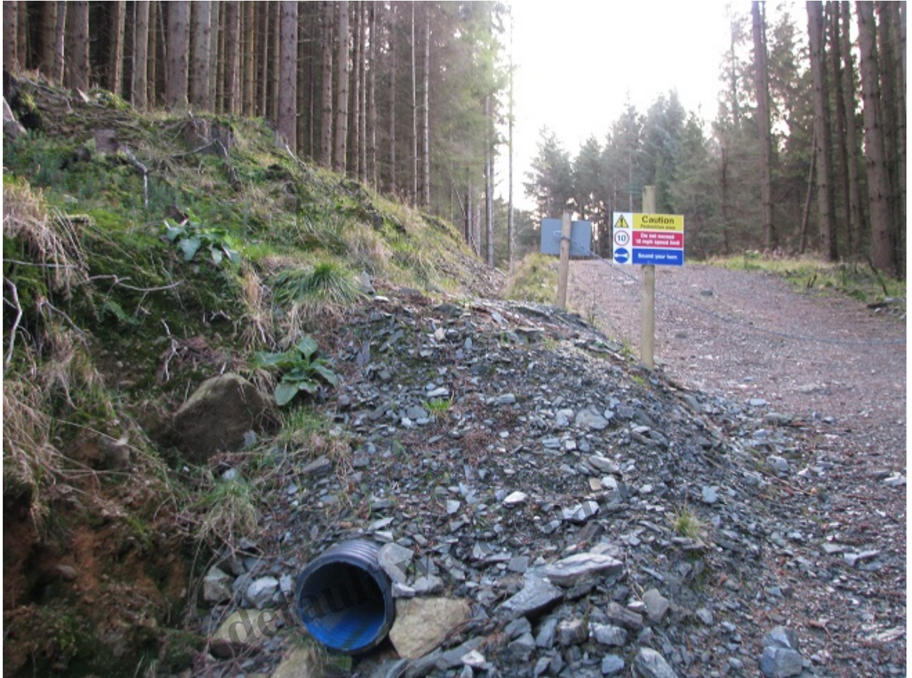
The poor finishing of culverts pictured here is evident in almost all the hydro scheme tracks in the Loch Lomond and Trossachs National Park. Photo Jane Meek.
