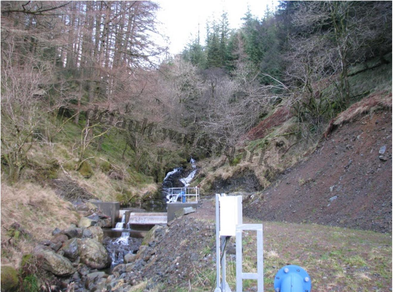
Ardchullarie hydro intake. While the intake is well located, nestling in the burn, the finishing contravenes the Loch Lomond National Park Planning Guidance on renewables: the intake dam is concrete and not finished with natural materials; the two intake vents are the usual Park blue whereas they should be in colours that match the natural landscape; the safety fencing on the intake again stands out and the slope on the right is an eyesore. Photo Jane Meek.
