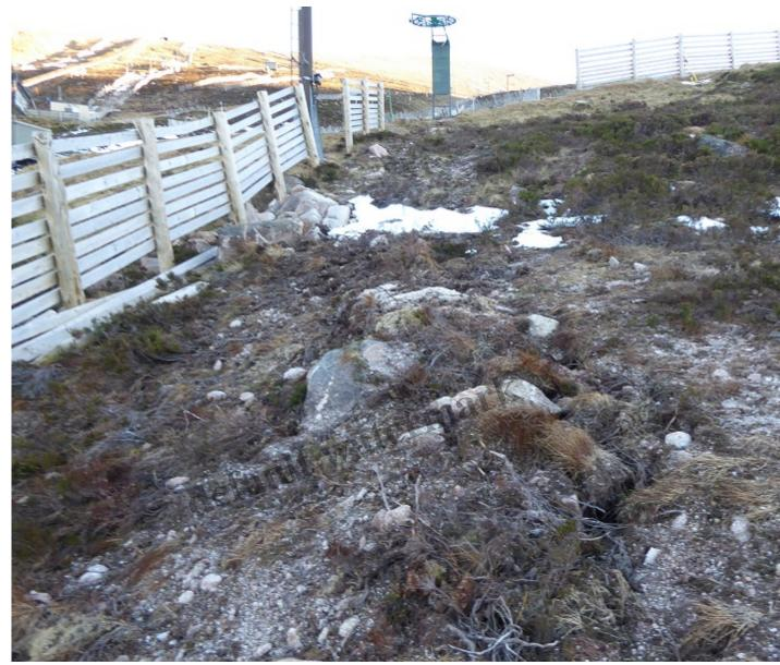
The poor "restoration" of the new car park t-bar cabling agreed by Highland Council on a de minimis Boulders have been dumped by the fence and the cable trench has not been properly filled in so a d has been created.
