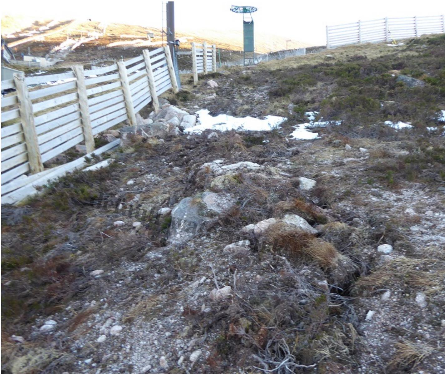
The poor “restoration” of the new car park t-bar cabling agreed by Highland Council on a de mi Boulders have been dumped by the fence and the cable trench has not been properly filled in so a d has been created.
