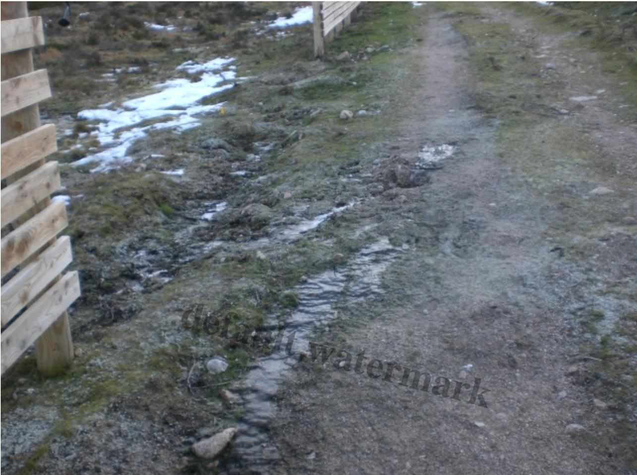
There was no sign of the hole, centre right, when I walked down the track two days before. Two days of freeze thaw and another section of track had been destroyed.
