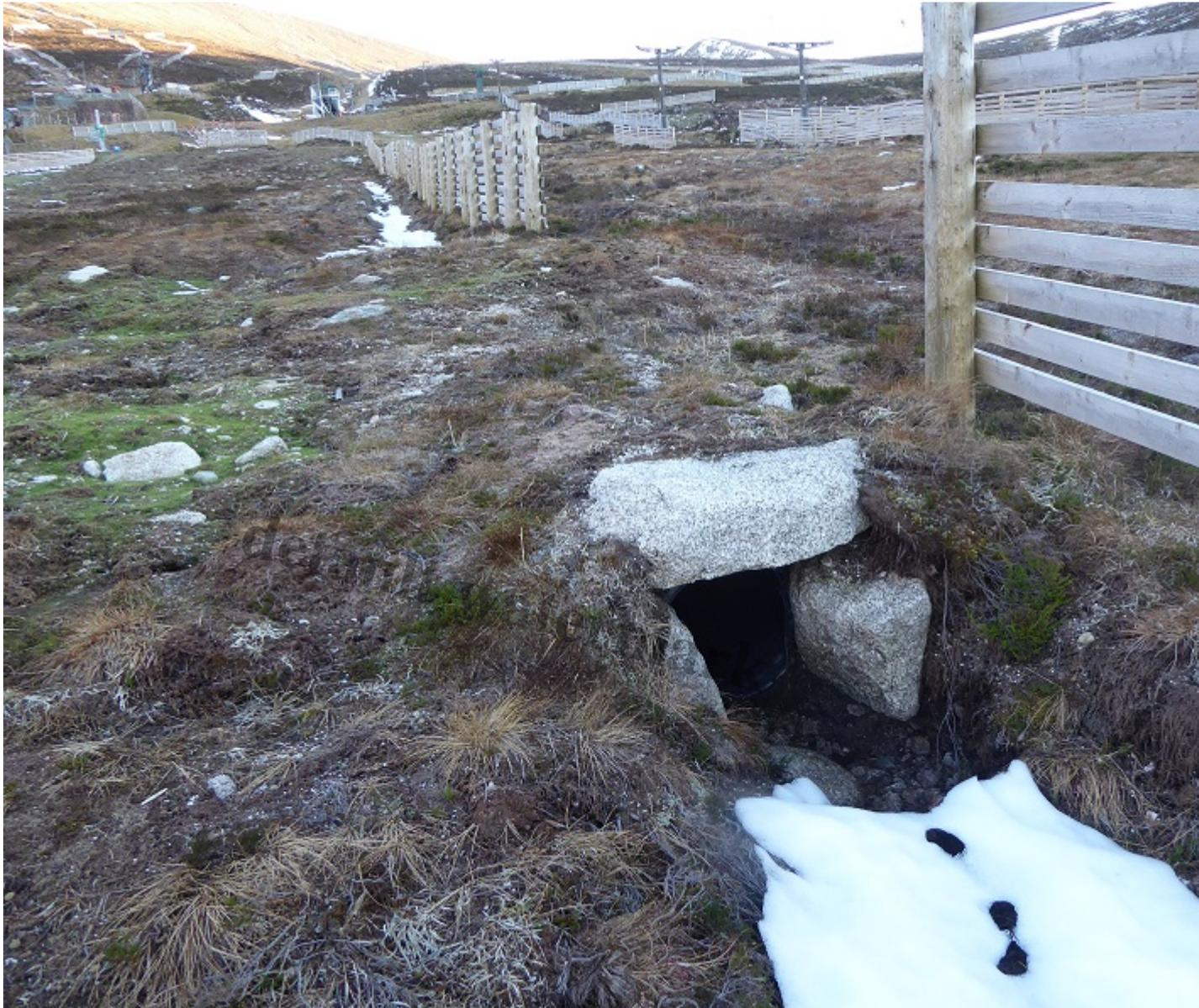
The seeding indicates that this culvert on right side of left shieling slope is new. The drainage line to fence is not mentioned in the Committee Report or accompanying papers.
