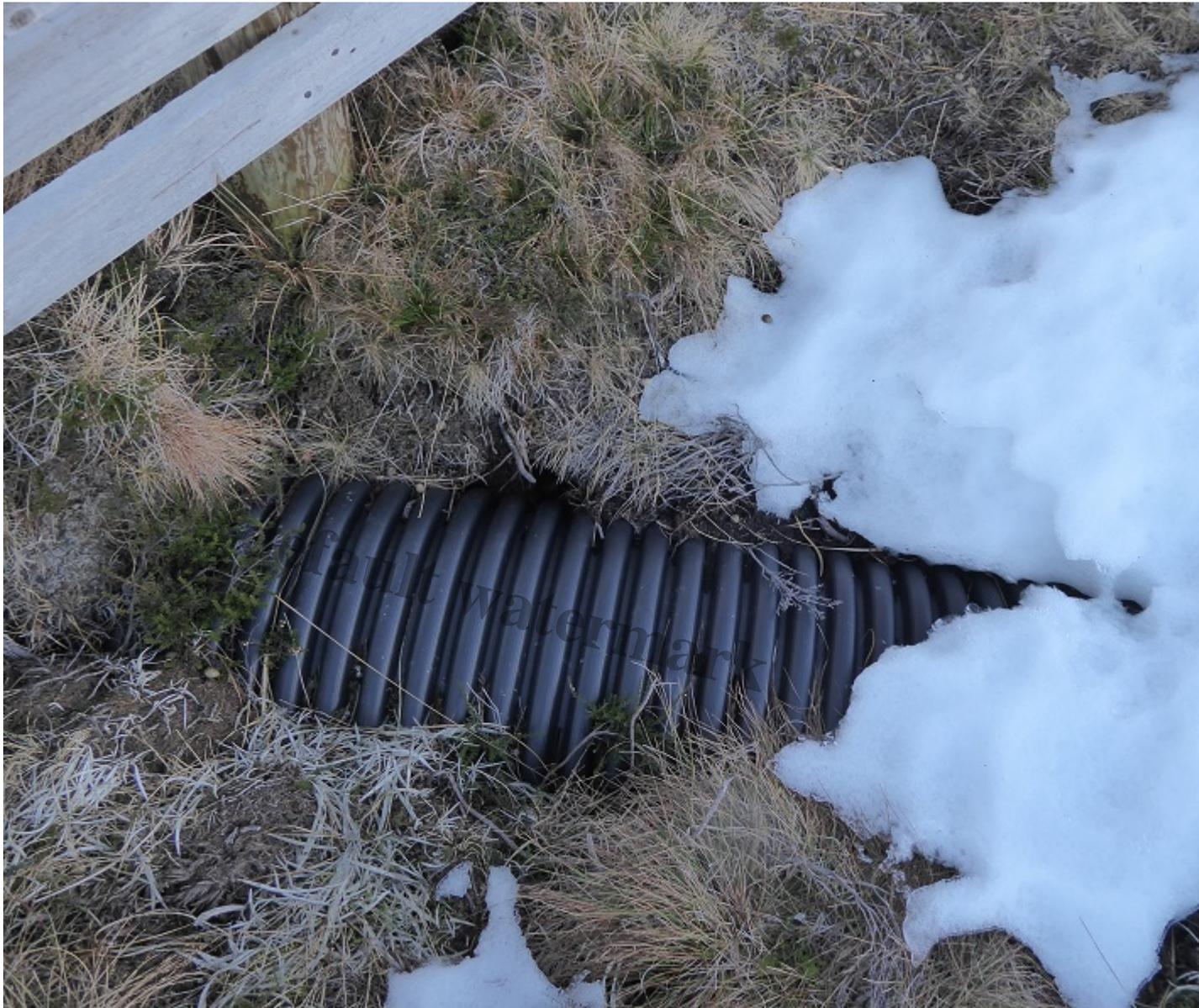
Section of poorly finished culvert crossing ski slope
