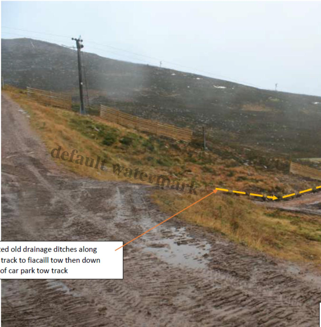
Reinstated old drainage ditches along existing track to fiacaill tow then down outside of car park tow track
