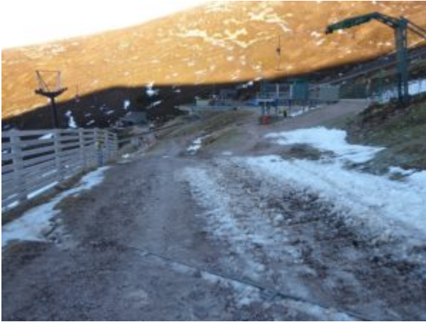
Choked steel drainage channel by Cas Gantry
