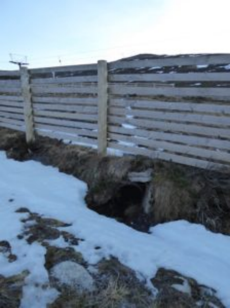
New? and poorly finished culvert at bottom of Shieling slope on left.
