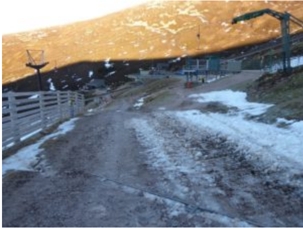
Choked steel drainage channel by Cas Gantry
