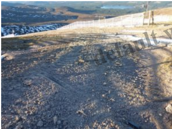
Choked drainage channel below Ptarmigan
