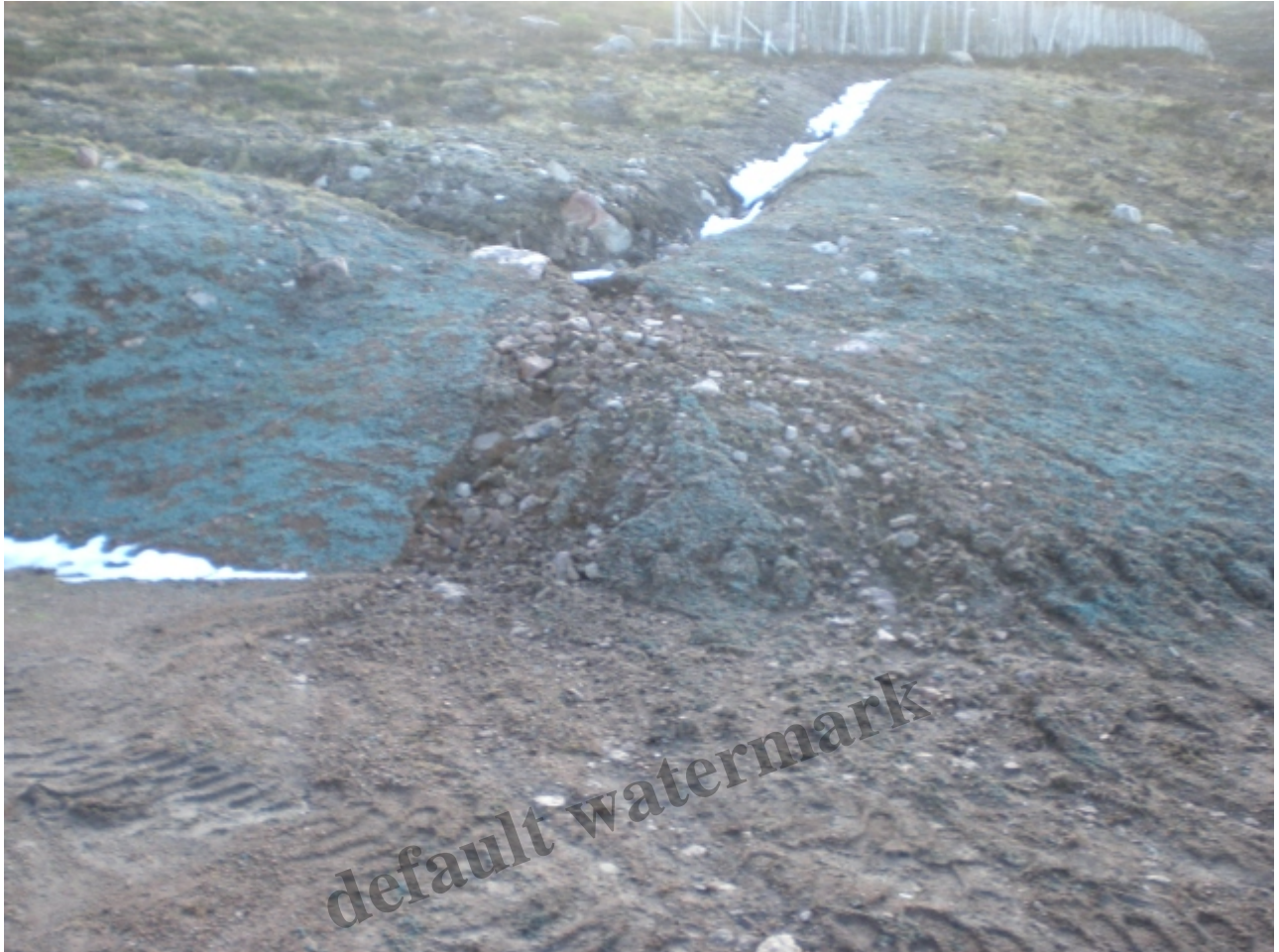
The ground to the right of the gantry, looking uphill showing where the blue revegetation pellets and topsoil have been washed away Photo Credit Alan Bratney 8/1/16
