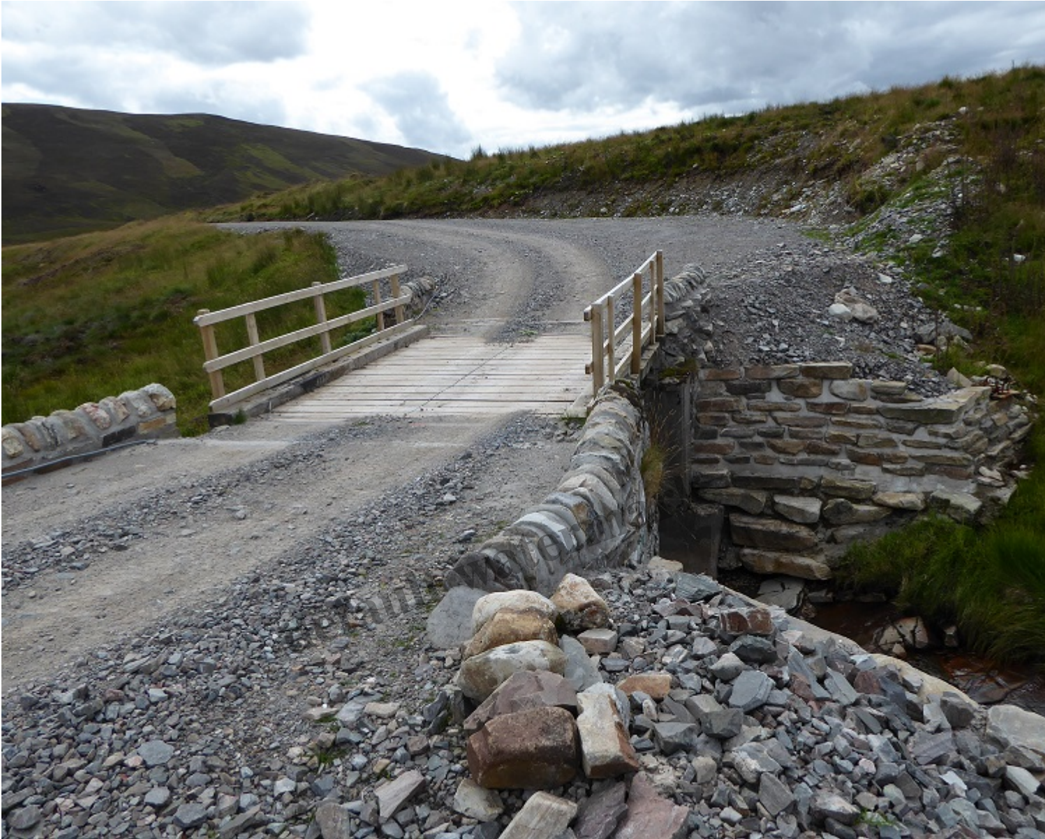
Another view of the not quite finished bridge
