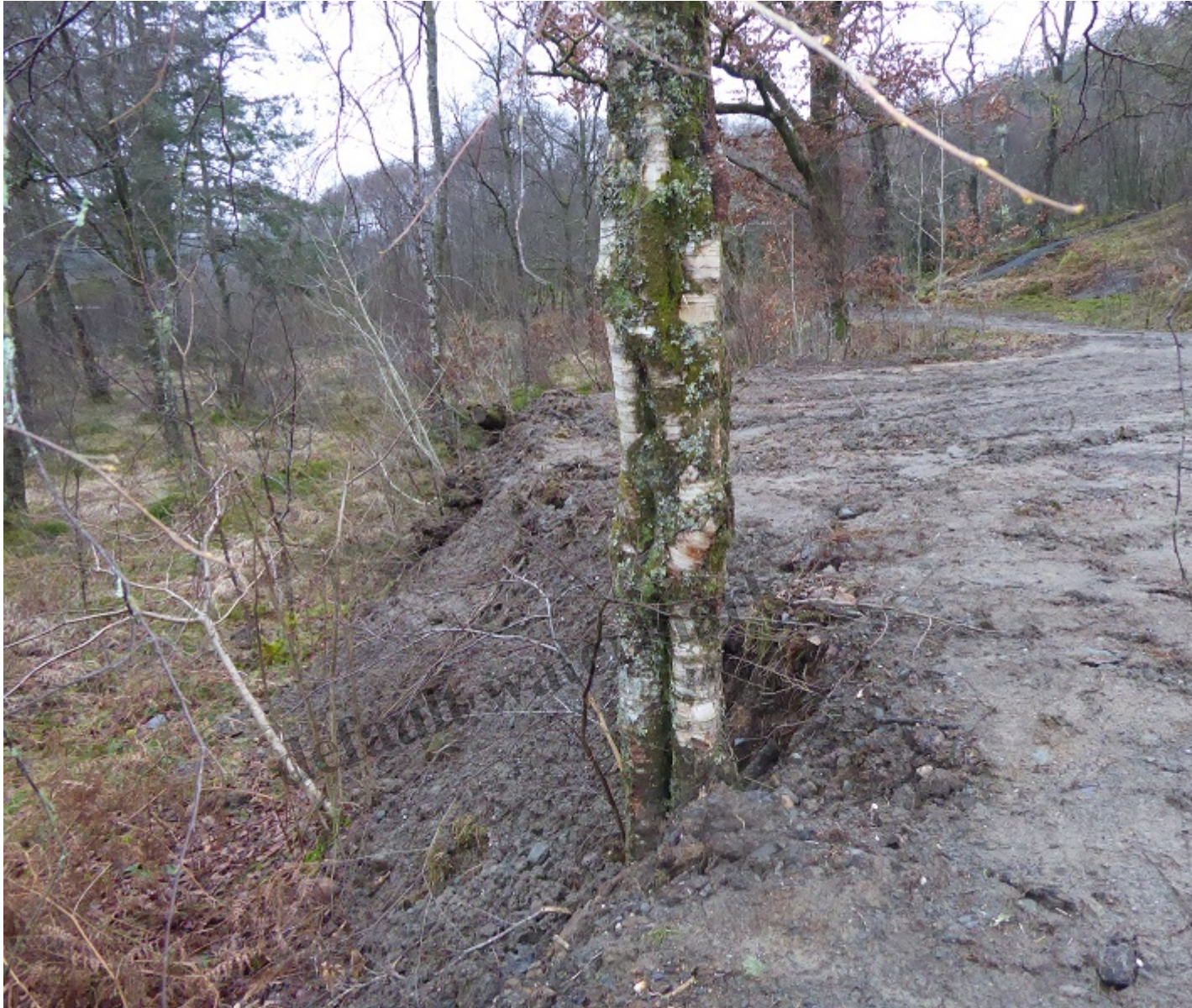
The new car parking area and site for toilets
