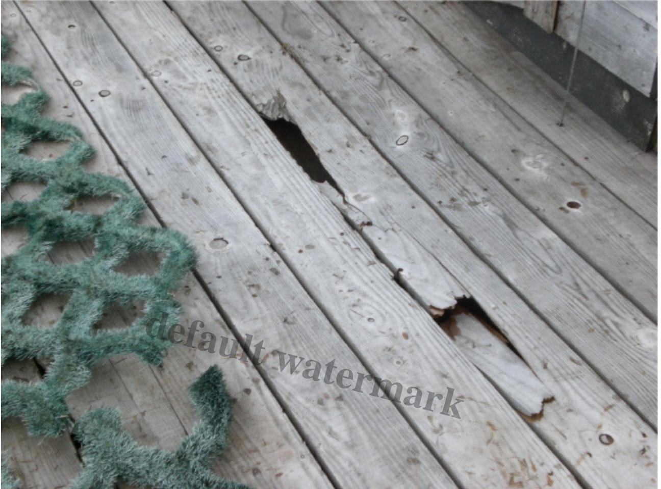
Loading ramp wood showing signs of rot
