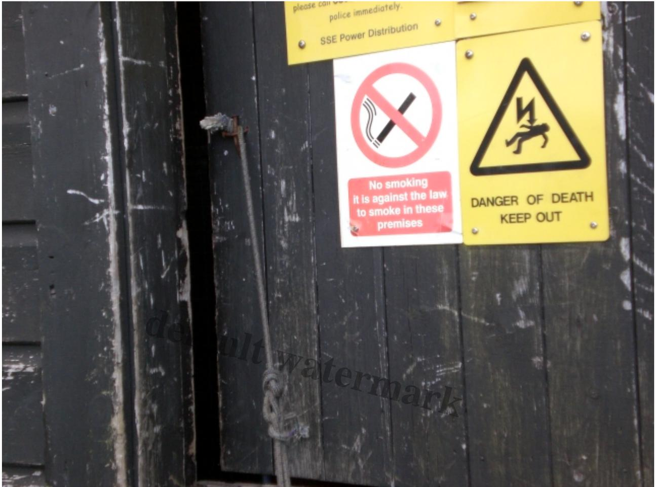
The control hut door does not close [tied together with twine but open enough to fill with snow in a storm.
