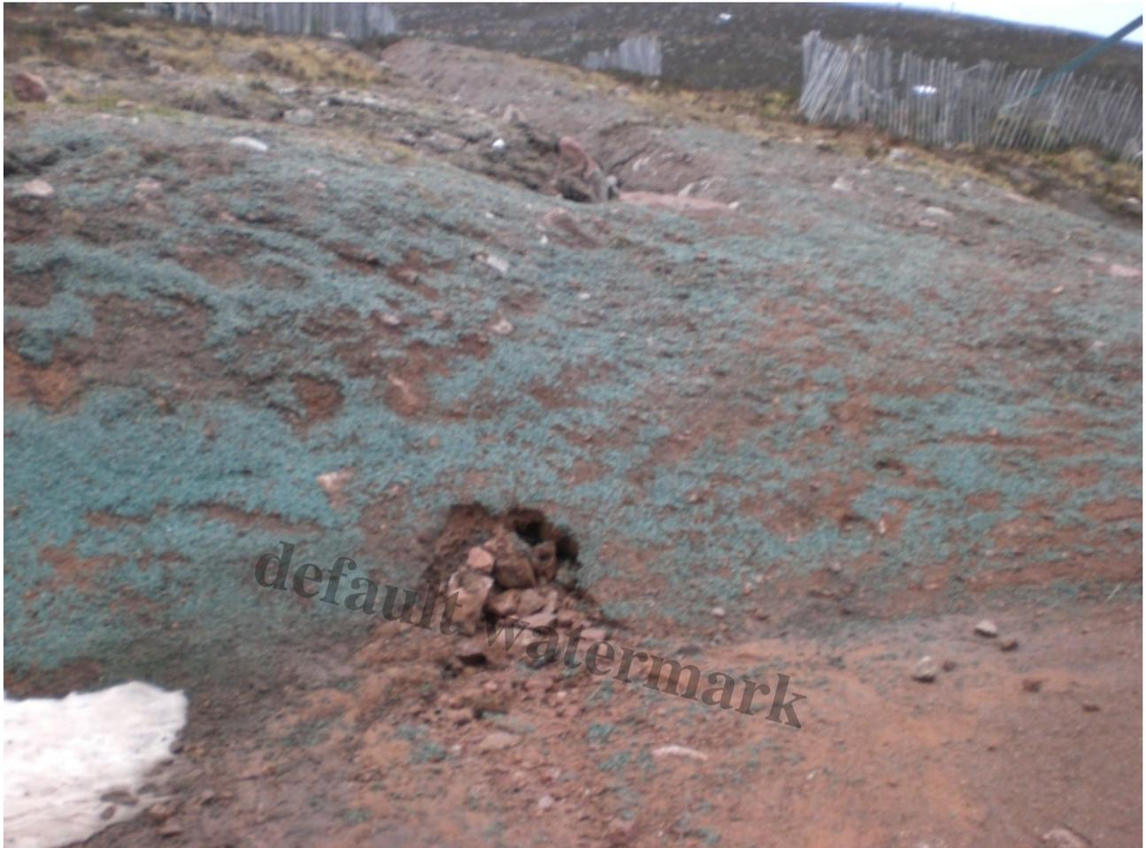
The “restoration” of the embanking. The blue reseeding pellets have been spread too late in the year and are being washed away by rainfall. You can see how the slope has begun to erode and its not difficult to predict that by the end of the winter the erosion will be far worse.
