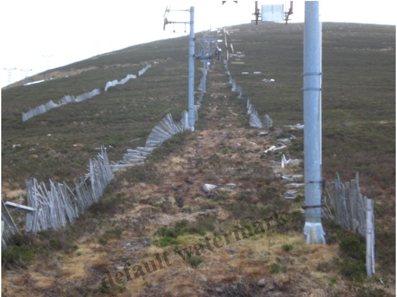
West Wall uptrack snow fencing December 2016 Photo credit Alan Bratney
