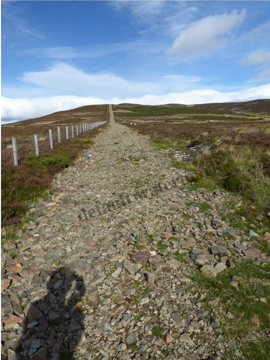
A closer view of track 1 from the start of the constructed section. The material for the track has simply been dumped on the moorland
