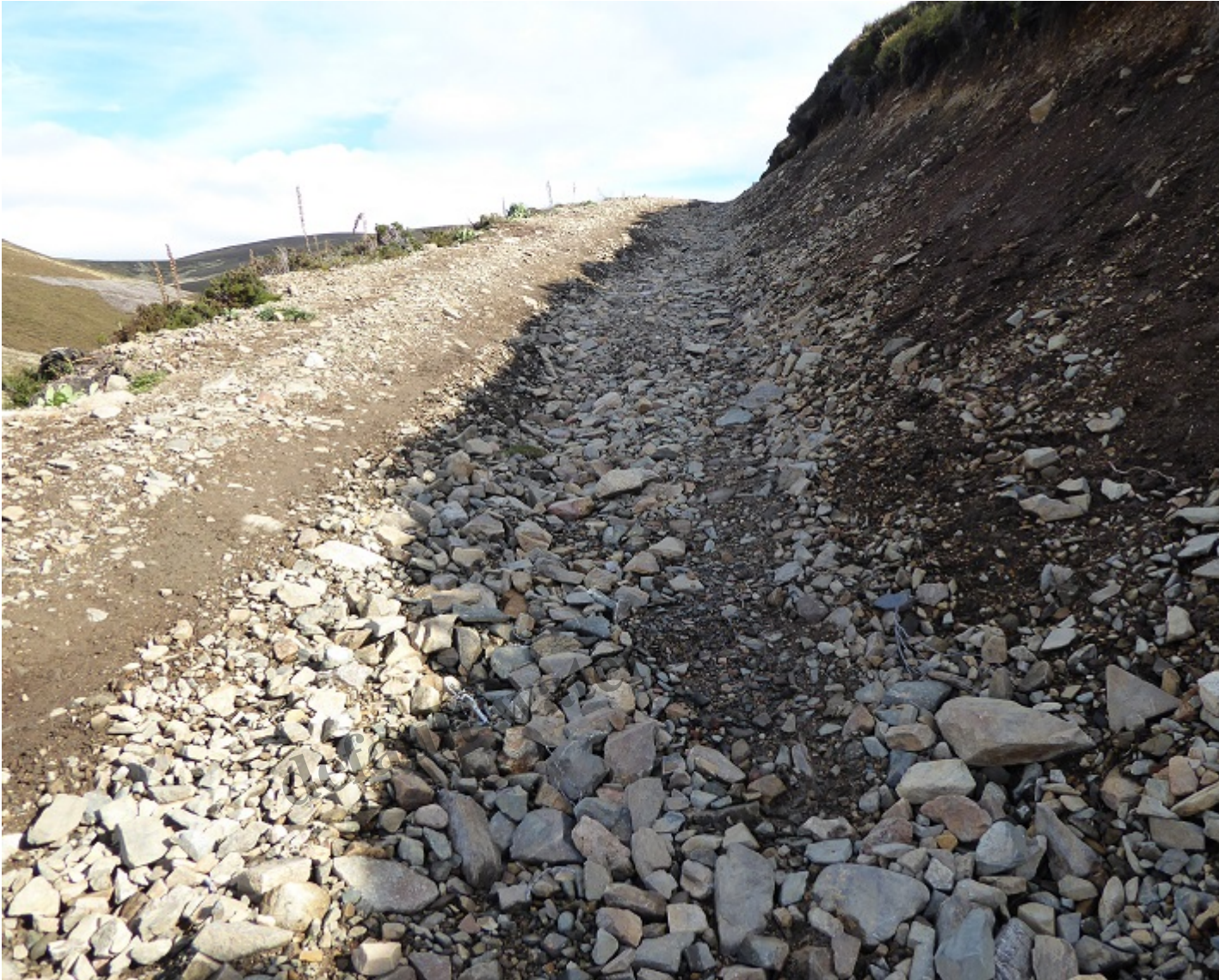
The eastern fork of track 2. The bank has been re-engineered and is too steep so vegetation is unlikely to recover and the track is also too steep.
