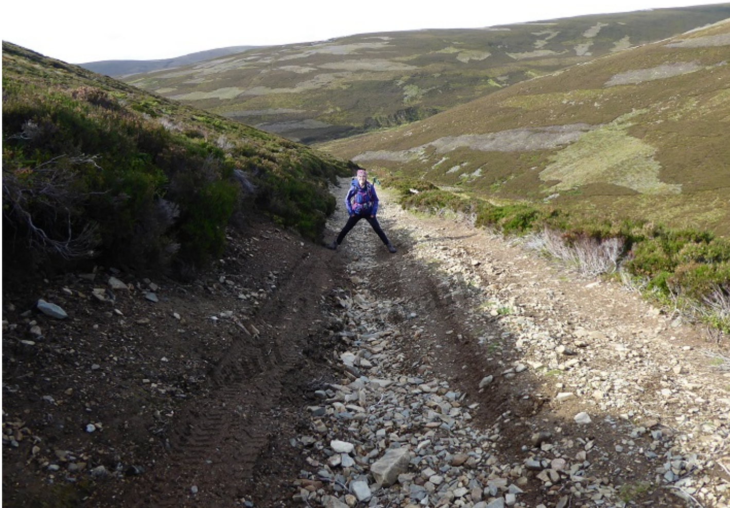
Gullying on track 2.
