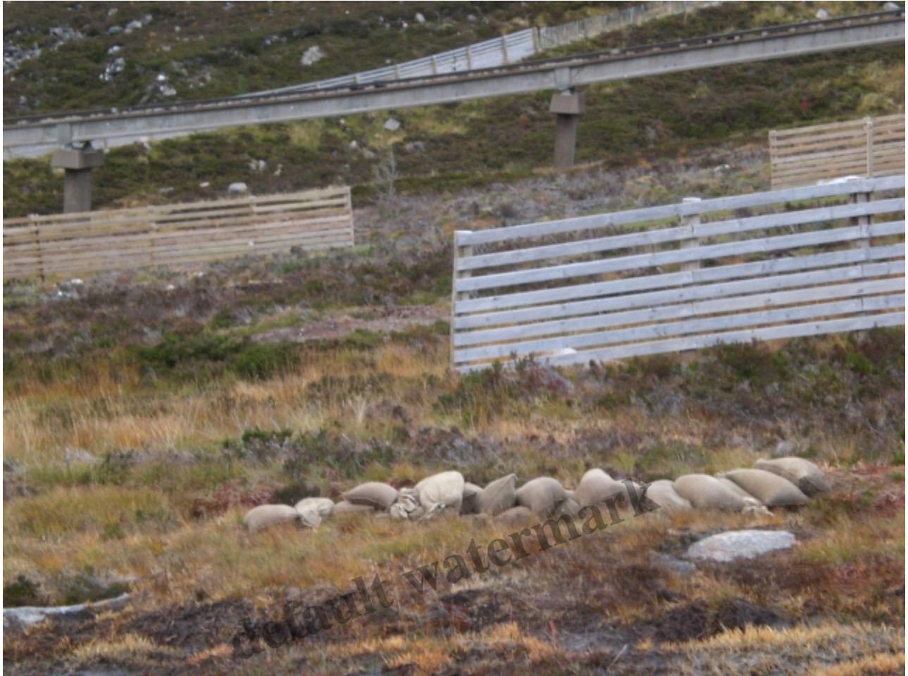
The unlawful Sheiling track runs in front of the middle fence while the rope tow runs behind it. Photo credit Alan Bratney
