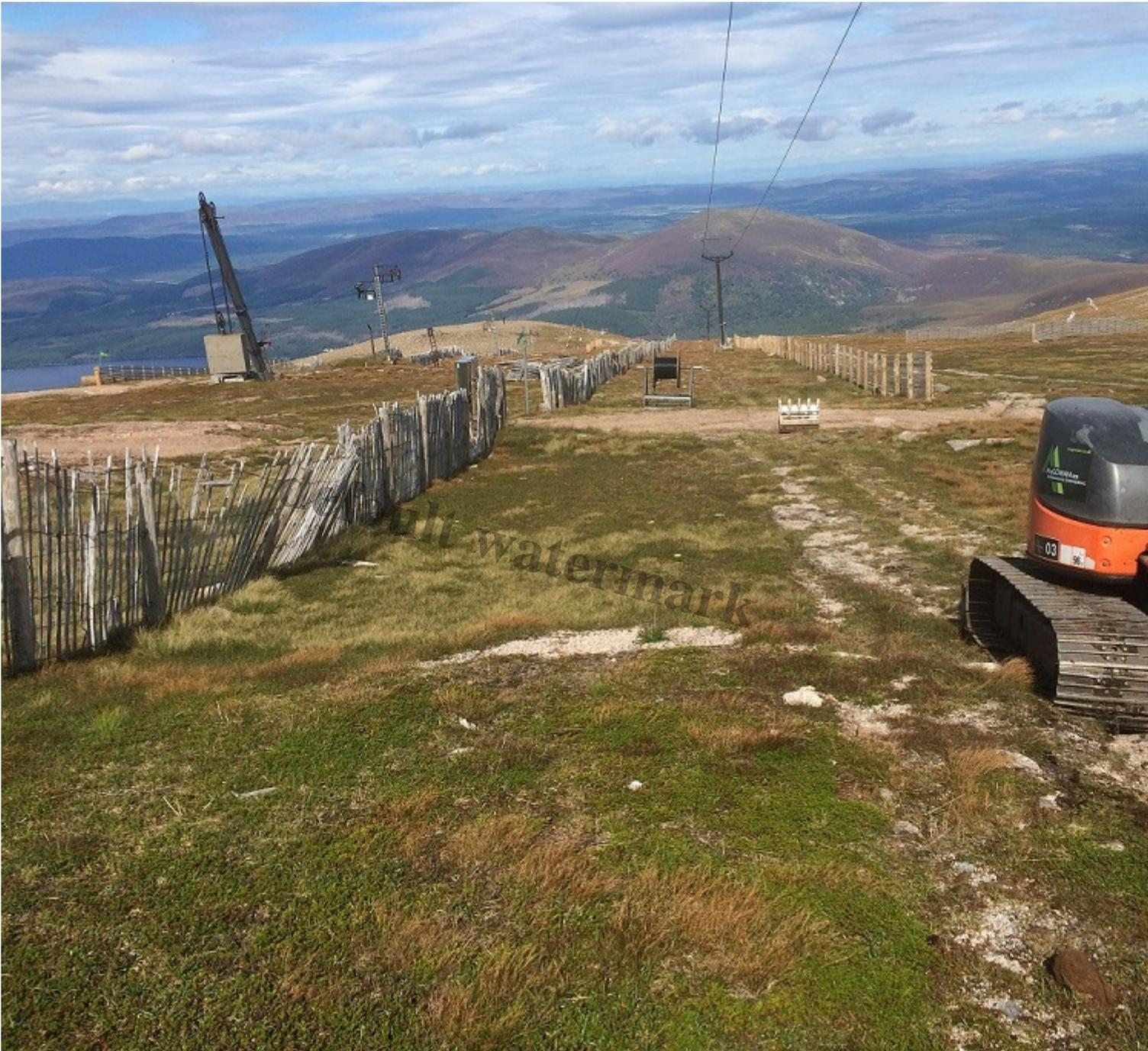
The caption to this read *Below you can see a digger starting work on the initial trench that that (sic) cable will go into. This ground will be fully reinstated once the entire cable is laid.*
