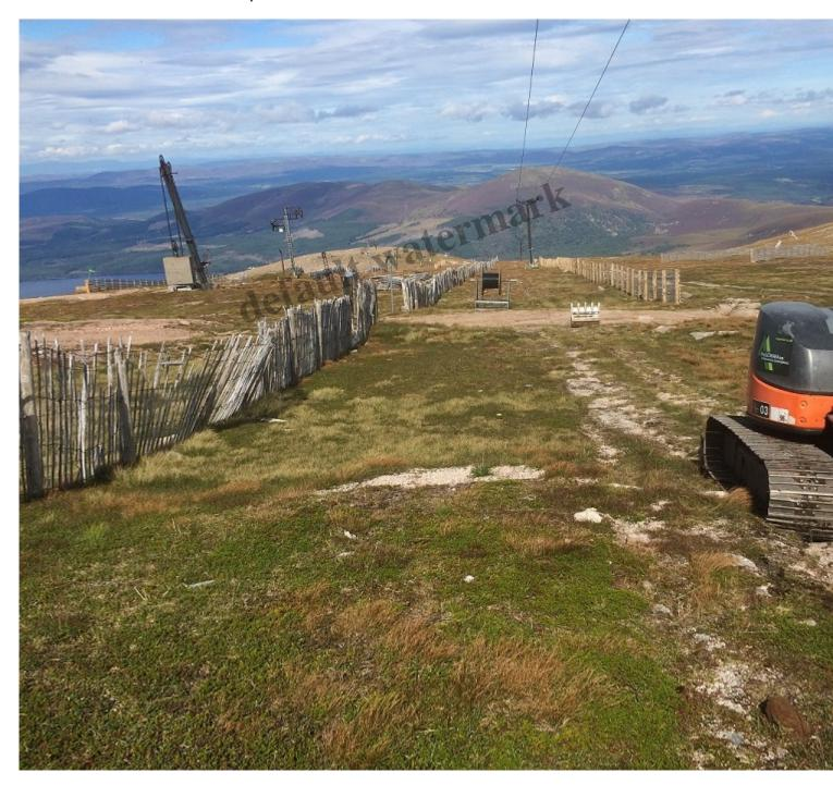
The caption to this read "Below you can see a digger starting work on the initial trench that (sic) cable will go into. This ground will be fully reinstated once the entire cable is laid."
