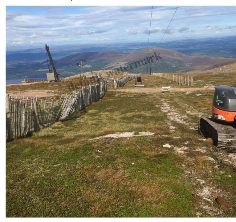
The caption to this read "Below you can see a digger starting work on the initial trench that that (sic) cable will go into. This ground will be fully reinstated once the entire cable is laid."
