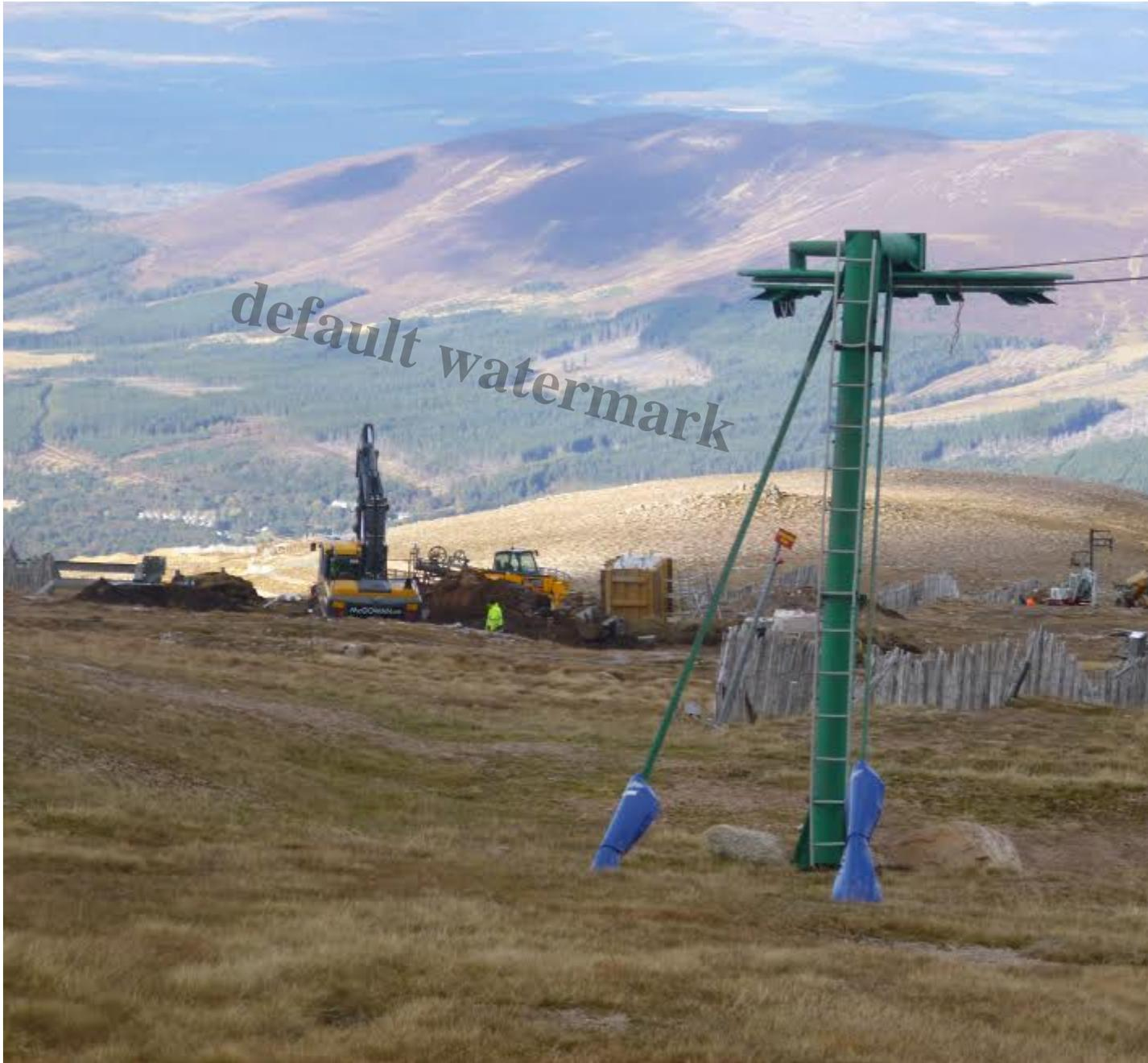
The new concrete plinth for the replacement West Wall poma return wheel can be seen just left of ce
