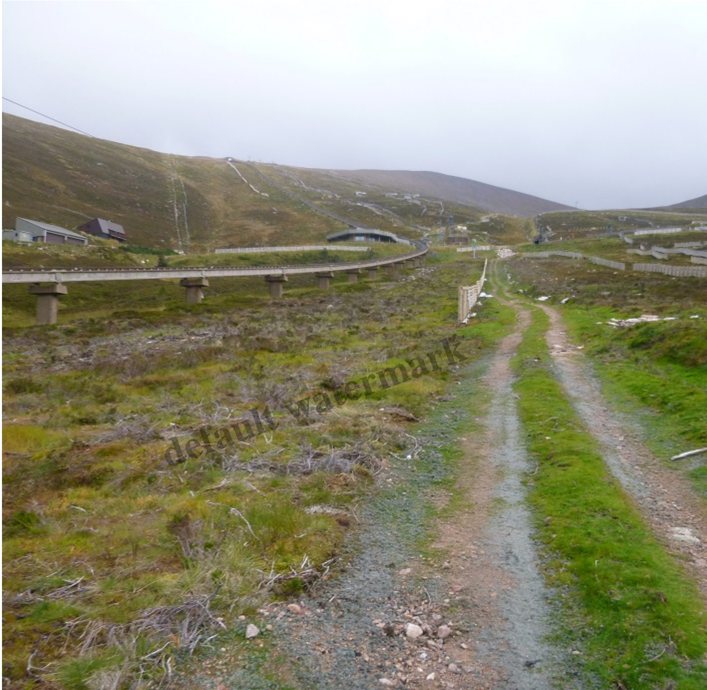
Half exposed pipes seem of no concern to the CNPA's landscape adviser
