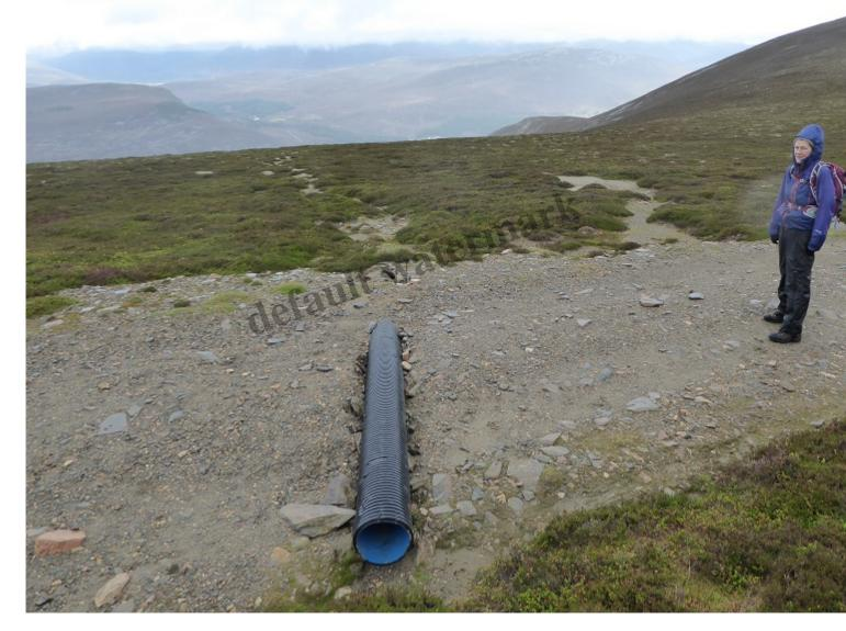
Standards of construction continue to be very poor. Behind the now useless drainage pipe, on the col below Morrone, you can see where material from the tracks has washed out over the moor.
