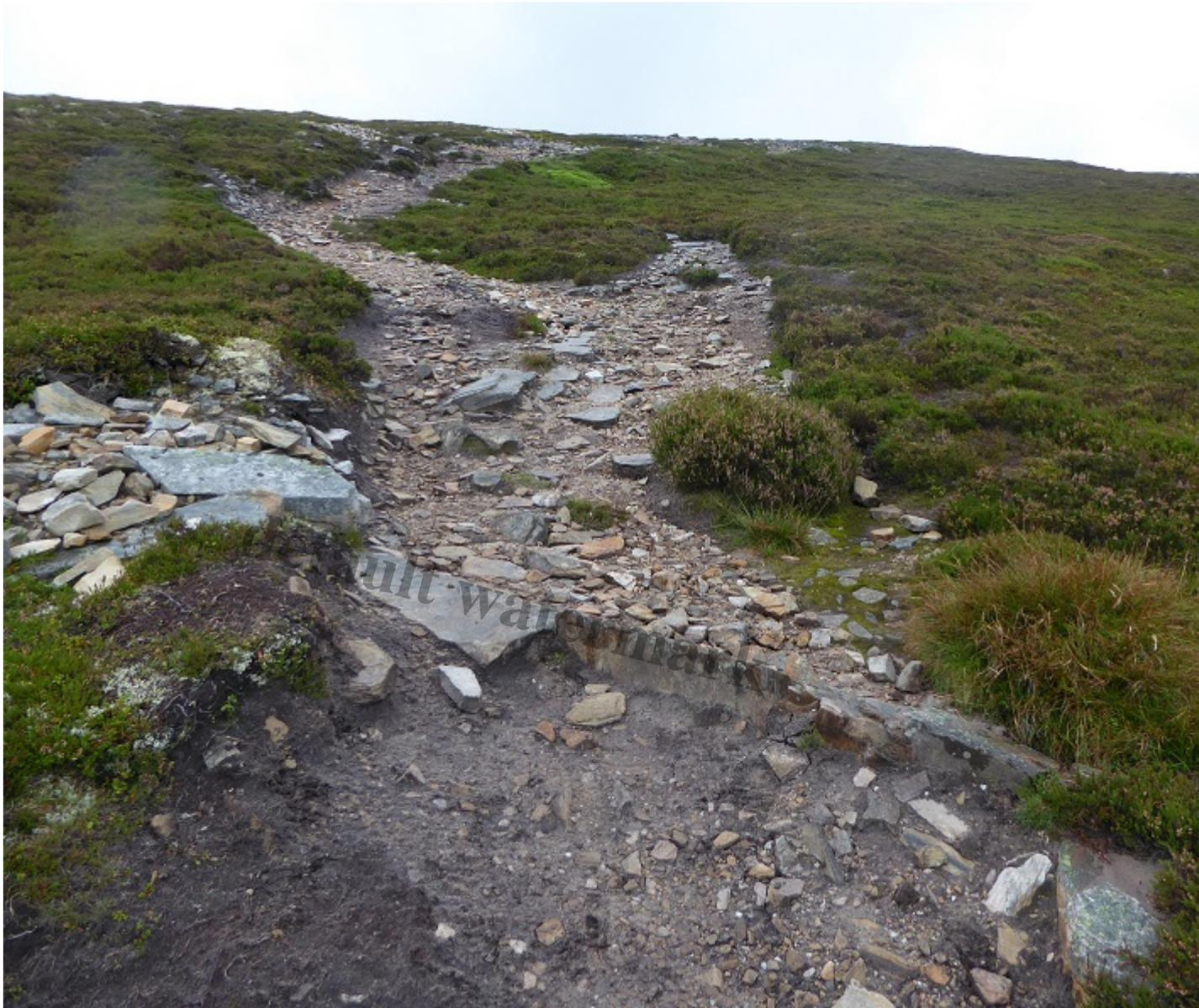
The broad erosion scar starts on the skyline where previous pathwork ended. This water bar needs work and was possibly never properly finished.
