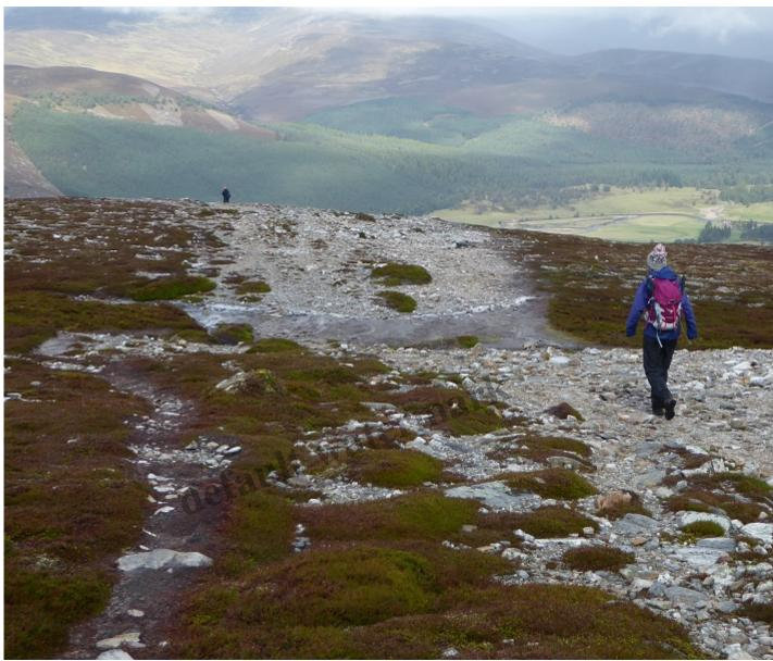
Top section of the Morrone hill path has been eroded by feet to create a broad scar that is still wider people take the vegetated ground on either side which is easier walking and less hard on the feet
