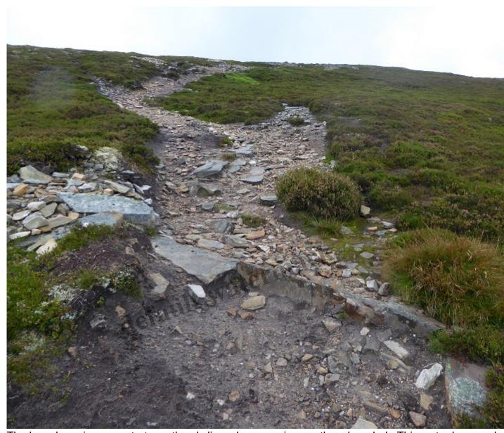
The broad erosion scar starts on the skyline where previous pathwork ended. This water bar needs further work and was possibly never properly finished.
