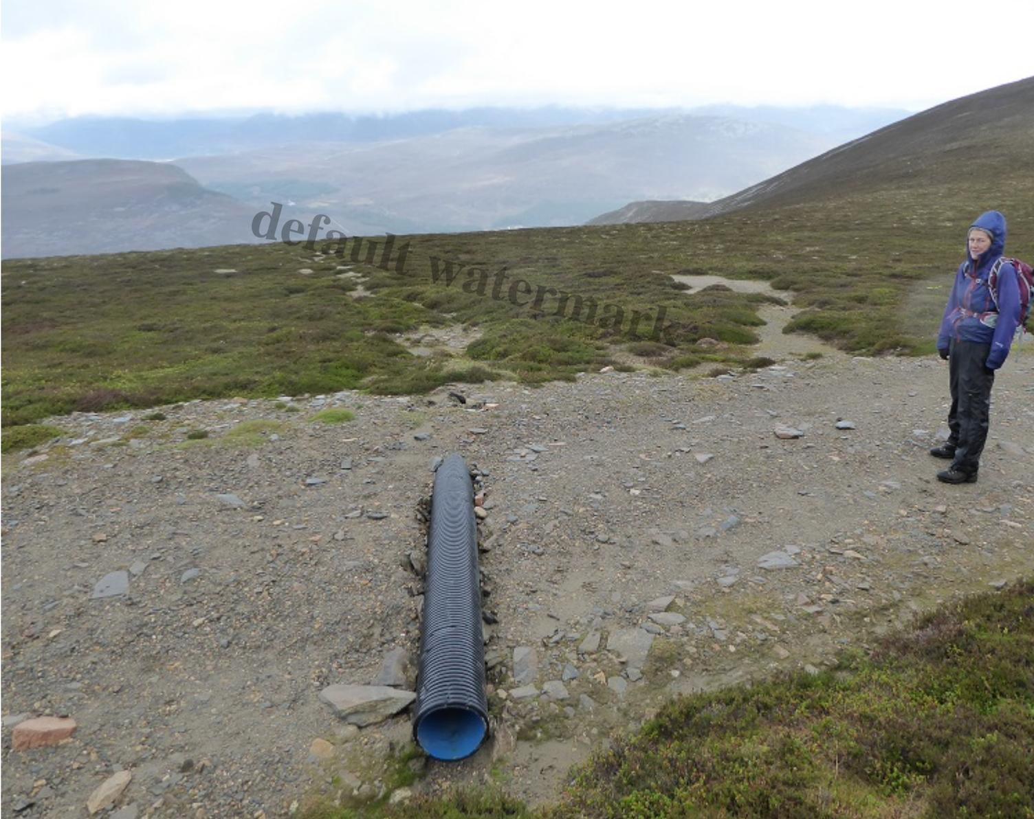
Standards of construction continue to be very poor. Behind the now useless drainage pipe, on the col below Morrone, you can see where material from the tracks has washed out over the moor.
