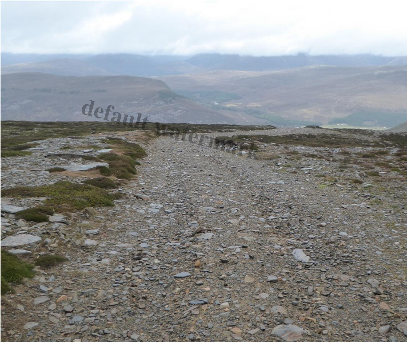
Morrone hill track. The track is extremely broad and neither the centre of the track nor the spoil which dumped on either side of it has re-vegetated (years after it was first bulldozed) increasing the visual
