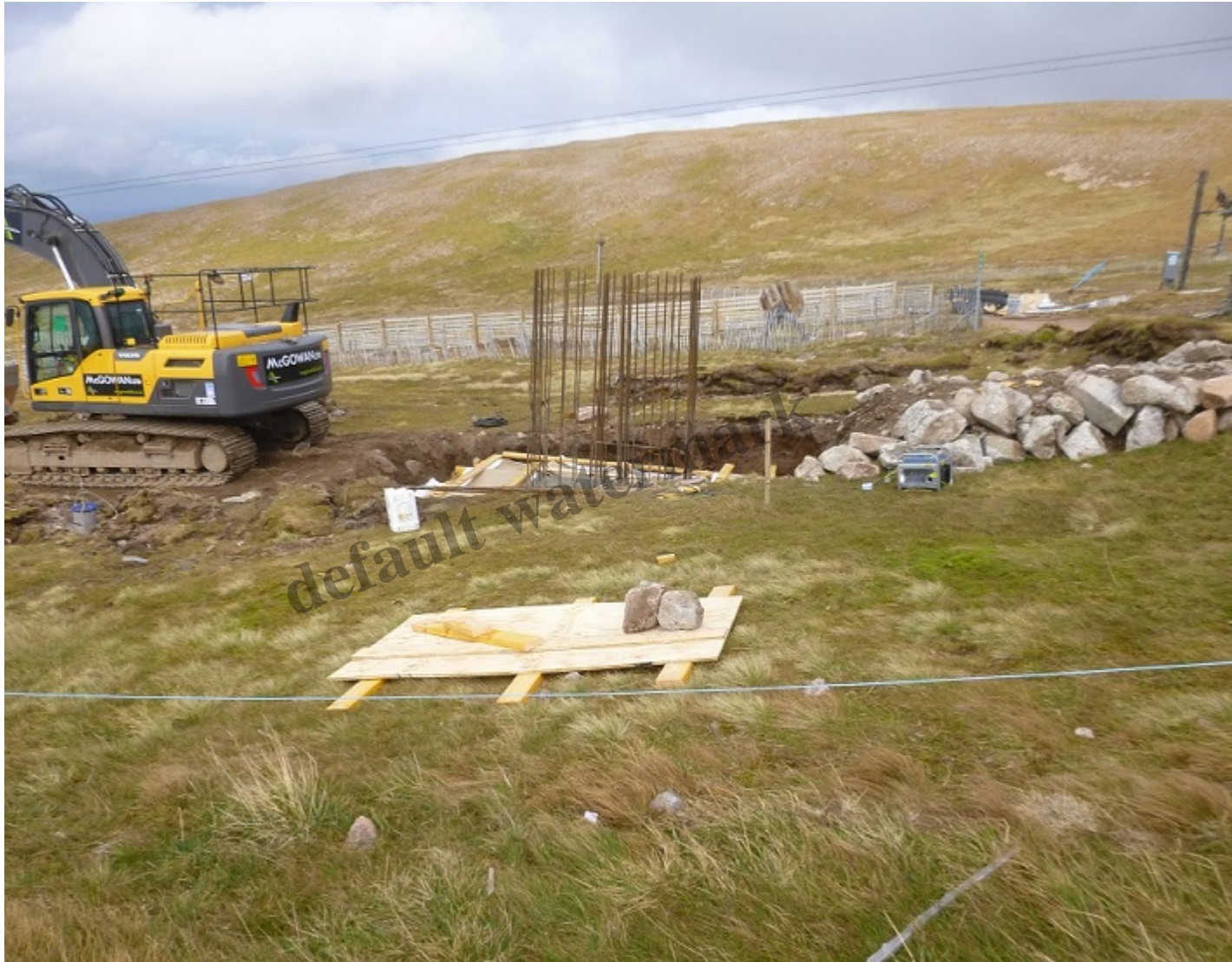
The foundations for the new fixed wheel at the top of the West Wall poma Photo credit Terry Smith
