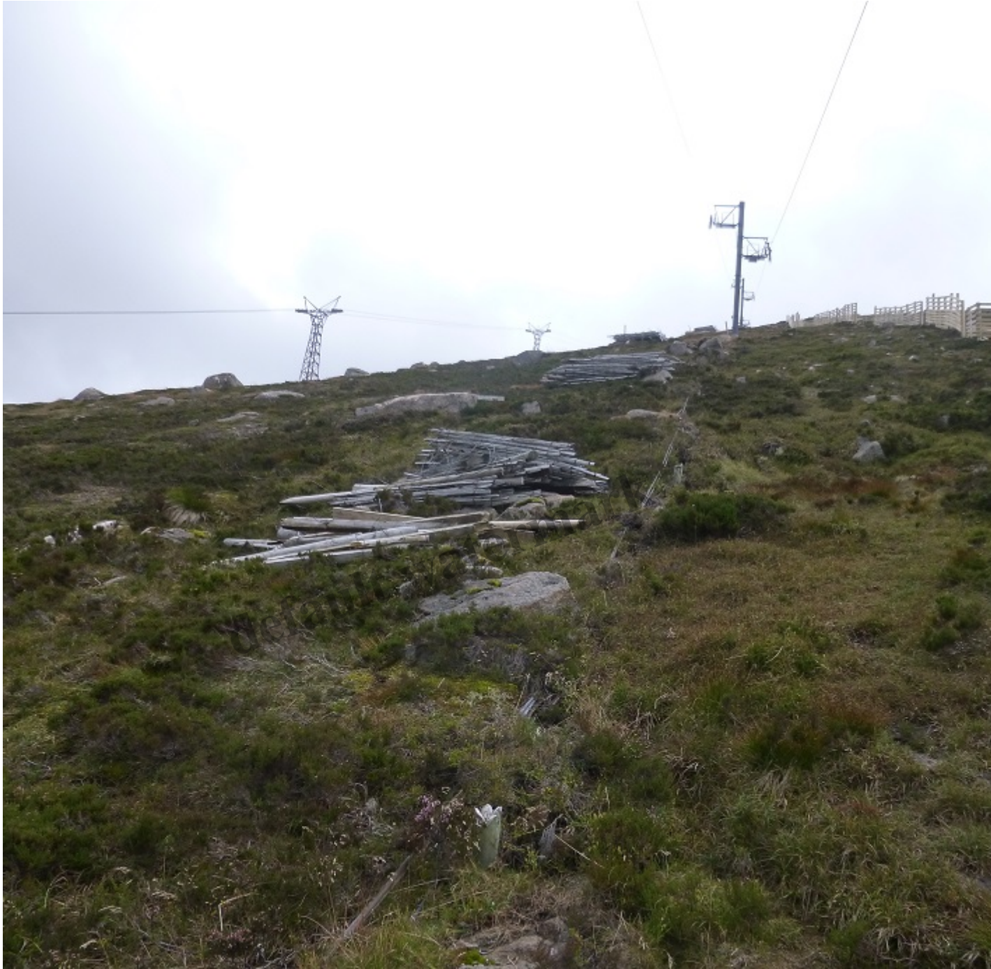
The old posts which supported the chestnut fencing have not been removed but simply broken off with an attempt to clear up old cabling
