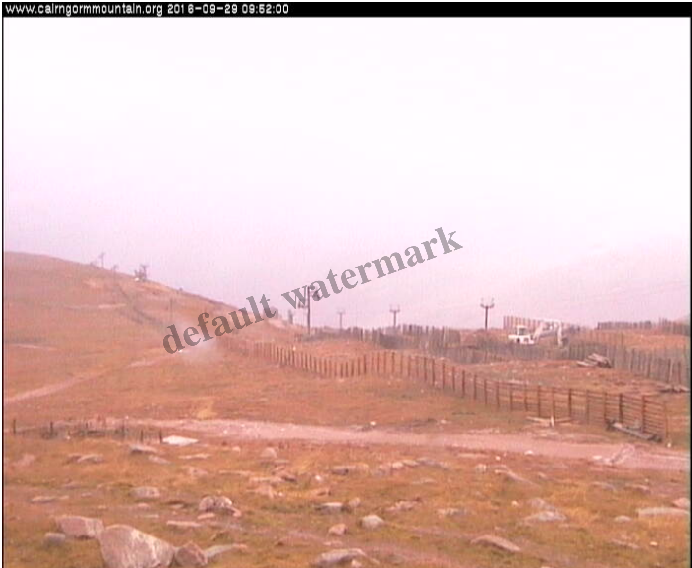
Digger operating outwith area granted planning permission – all vehicles were meant to be carefully controlled Photo from Cairngorm Mountain webcam (thanks to George Paton)
