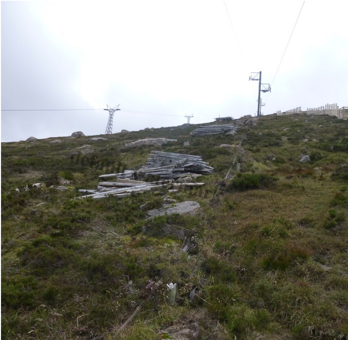
The old posts which supported the chestnut fencing have not been removed but simply broken off with a chainsaw to clear up old cabling
