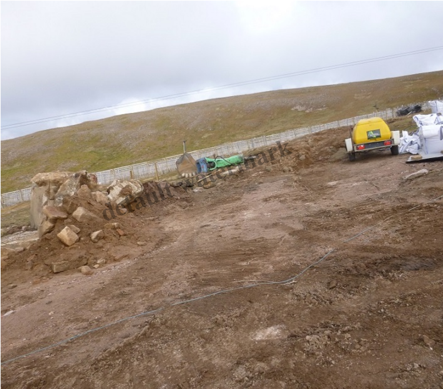
The building site near the top of the West Wall poma – Photo Credit Terry Smith 23/9/16
