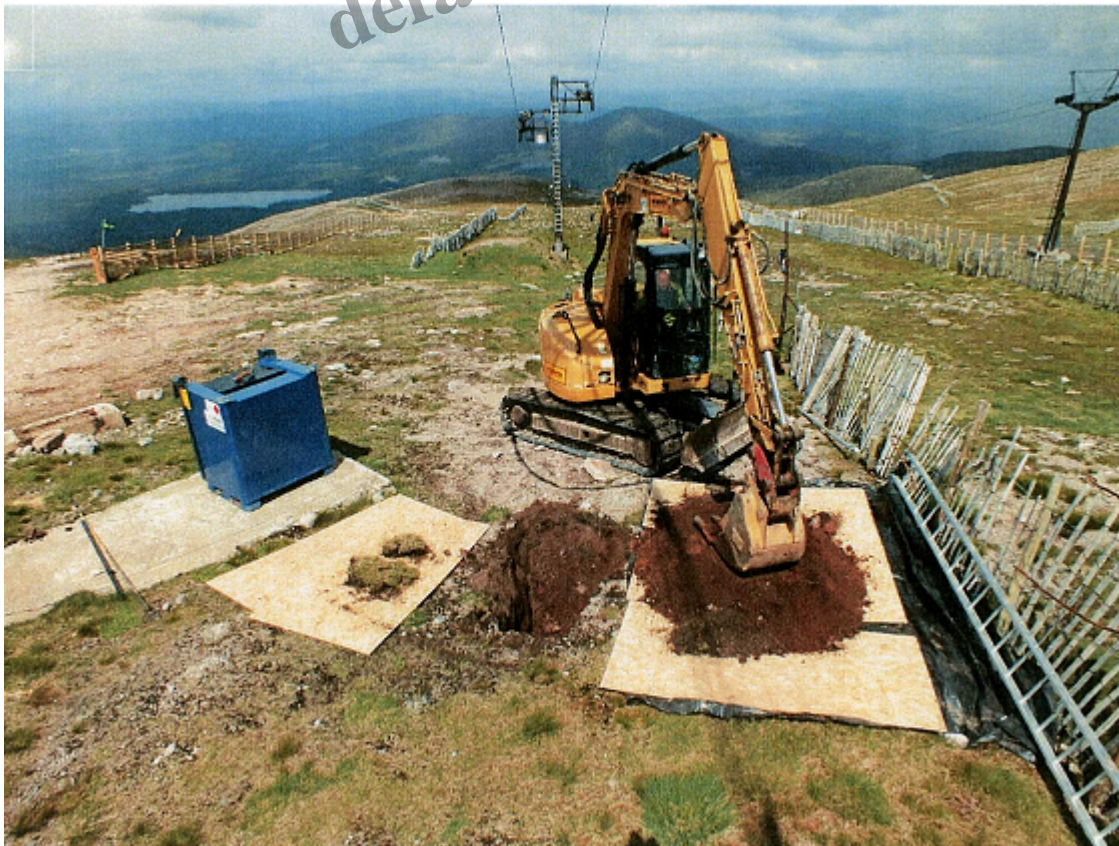
Note the use of the matting to protect vegetation – photo from ADAC report.
