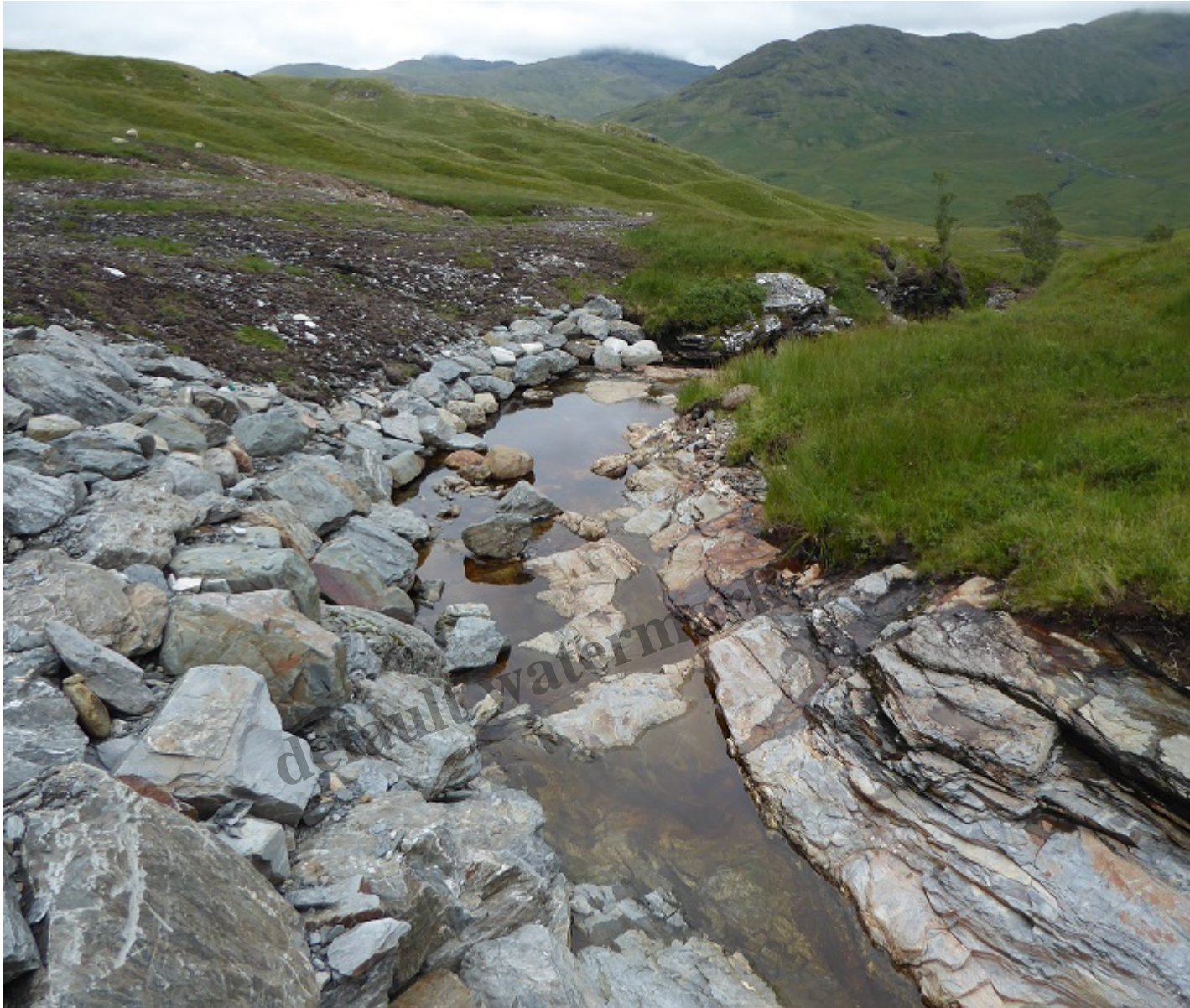
Rip Rap retention on Eas Eonan contrasts with the natural gorge below
