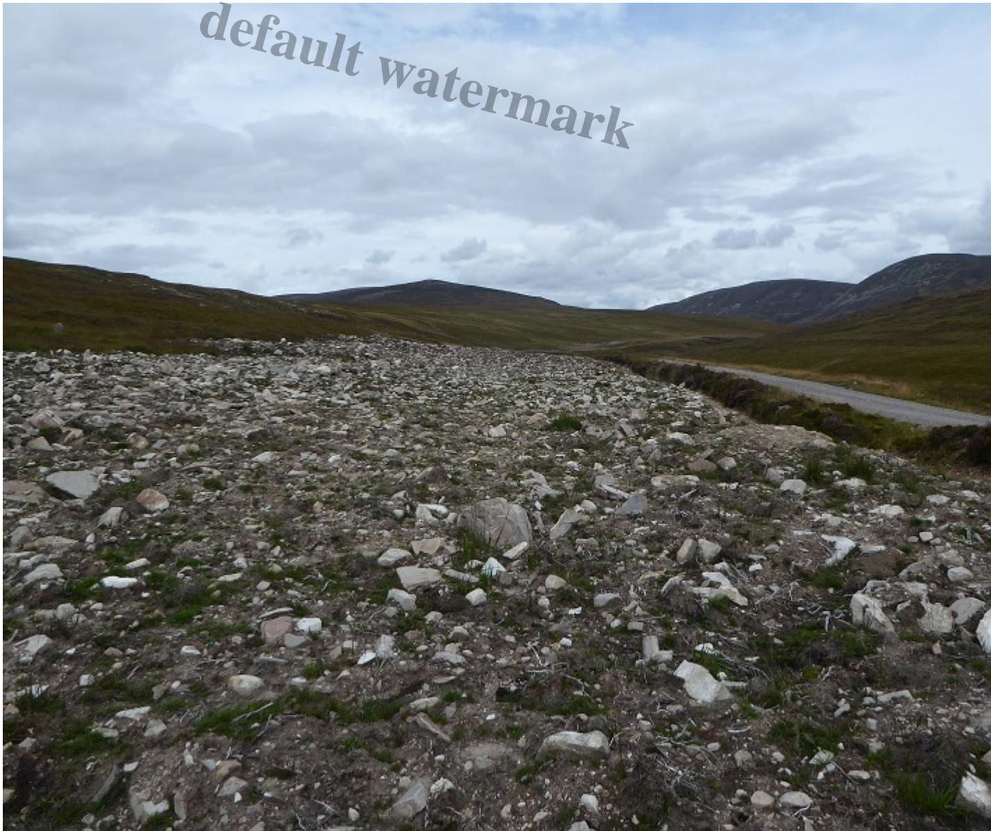
Destruction of moorland along the buried hydro scheme pipeline in Glen Bruar. There has been no a preserve the peat/topsoil and instead boulders/minerals have been left on the surface creating new s
