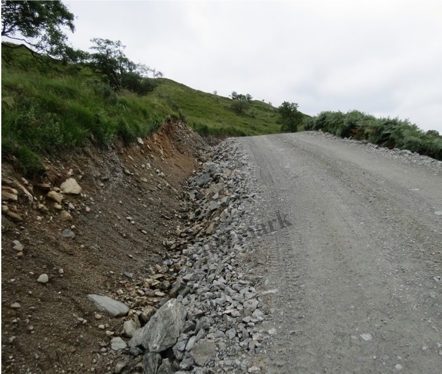
Part of the lower section of the access track to Ben Glas hydro scheme Glen Falloch illustrating the large amount of aggregate used in its construction
