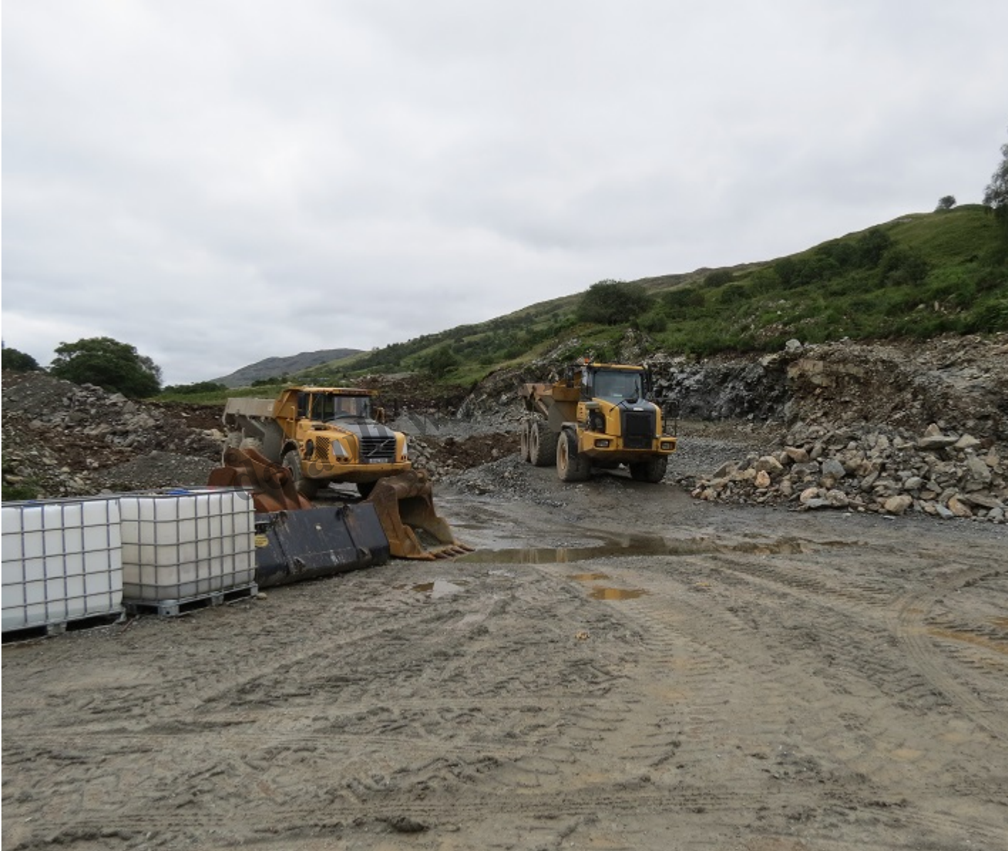
The quarry site at the bottom of new Ben Glas track
