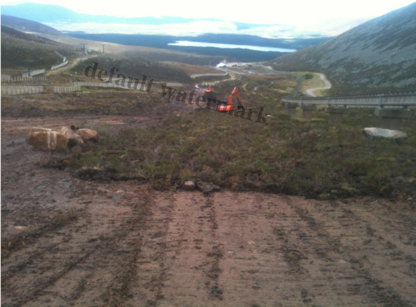
Image showing reinstatement of turf on new ground contours prior to lift installation Oct 2015. Track on left of work site retained to move materials and ski lift components avoiding tracking on reinstated vegetation.
