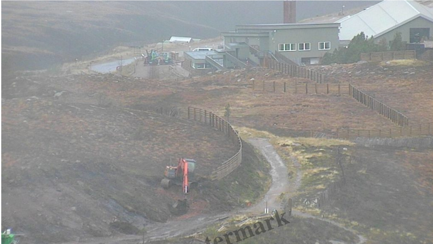
Destruction of the bank – photo credit Cairngorm Mountain webcam
