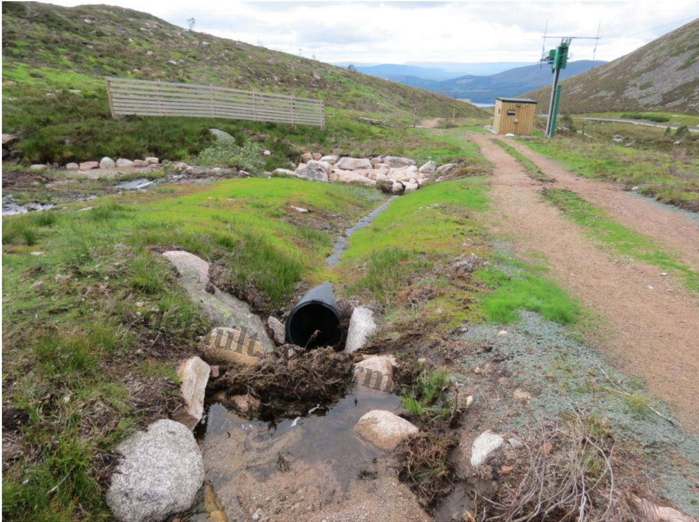
One of two unfinished culvert on the edge of the Sheiling Poma ski slope – there are three culverts in all, only two of which are referred to in the planning application
