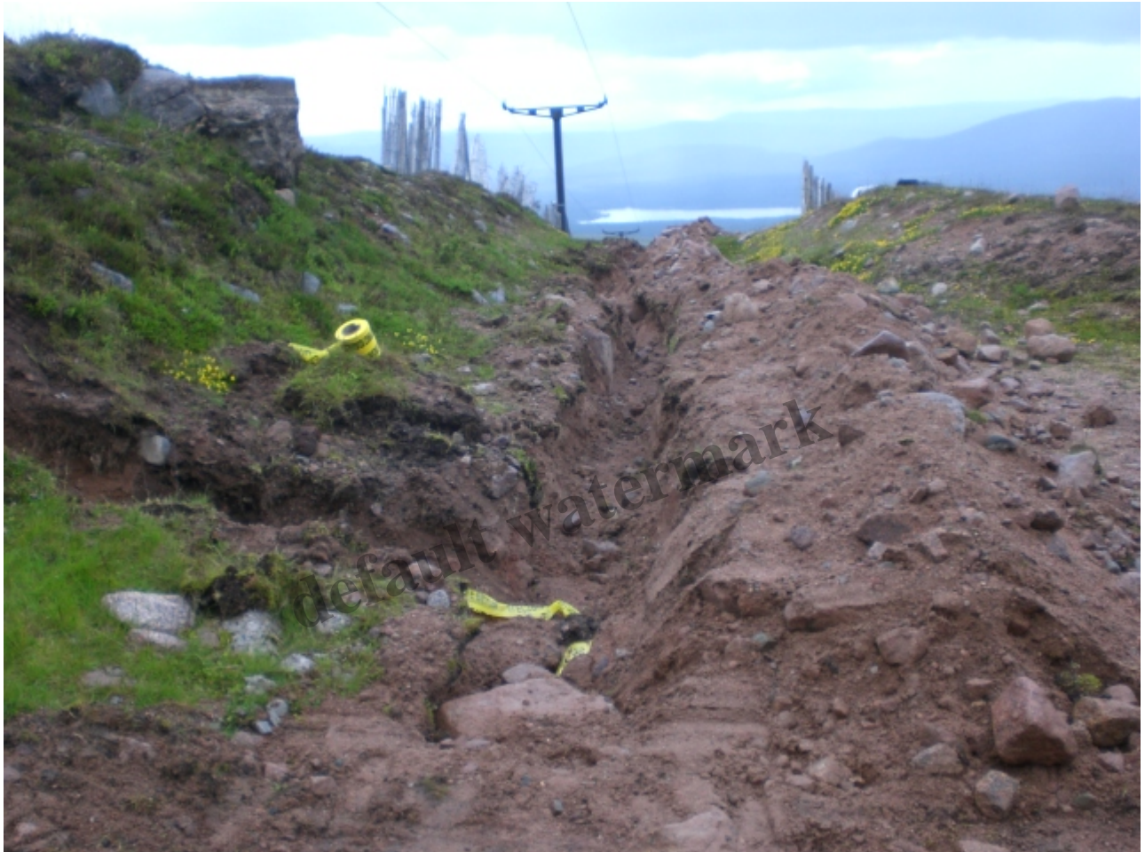
The trench that has been dug along the entire length of the car park T bar to install new cabling – photo credit George Paton
