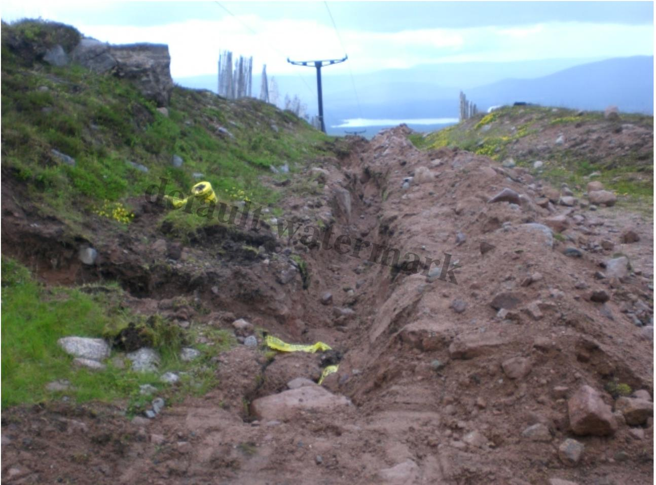
The trench that has been dug along the entire length of the car park T bar to install new cabling â?? photo credit George Paton
