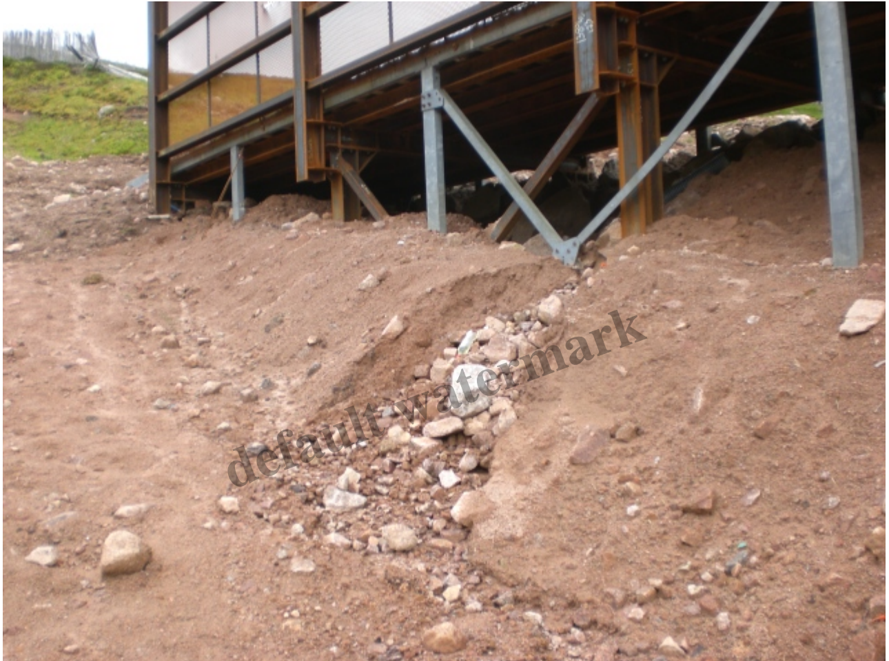
The new Coire Cas T-bar platform with spoil below. It is already being eroded away by the rain. Photo Credit Alan Bratney
