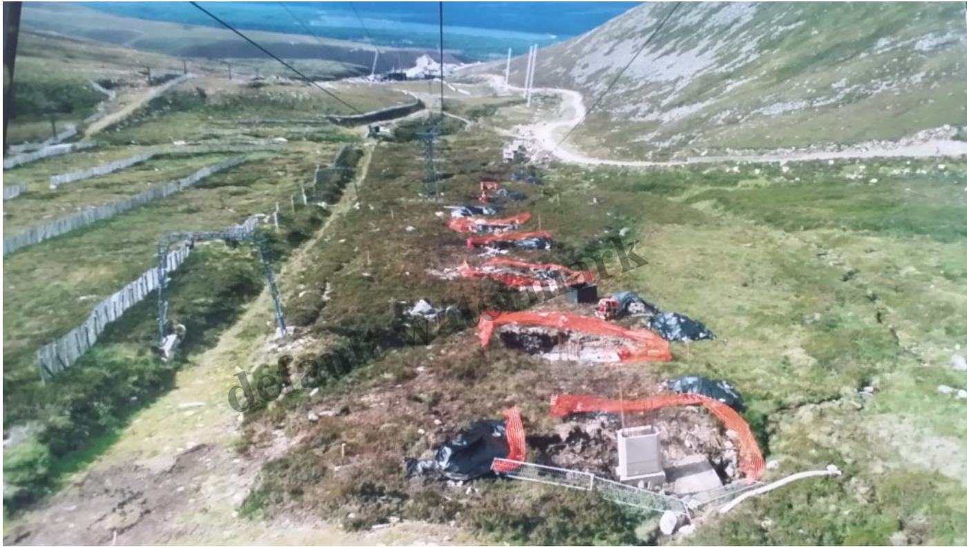
Funicular construction – Photo credit George Paton
