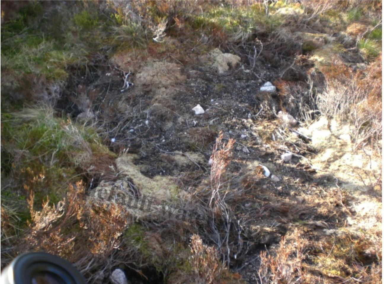
A hole excavated by a digger outwith the area granted planning permission â?? it appears the contractors were short of vegetation (implying they had not stored turf in the manner specified) and tried to address this failure by taking vegetation from elsewhere. There is no mention of this in the Method Statement and it is also clearly outwith the planning permission granted
