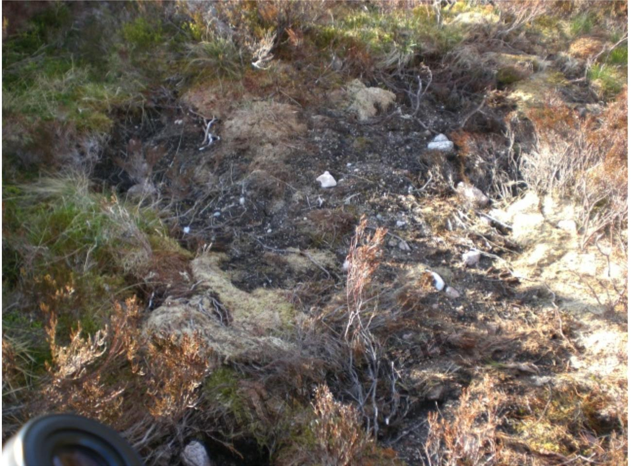
A hole excavated by a digger outwith the area granted planning permission – it appears the contractors were short of vegetation (implying they had not stored turf in the manner specified) and tried to address this failure by taking vegetation from elsewhere. There is no mention of this in the Method Statement and it is also clearly outwith the planning permission granted
