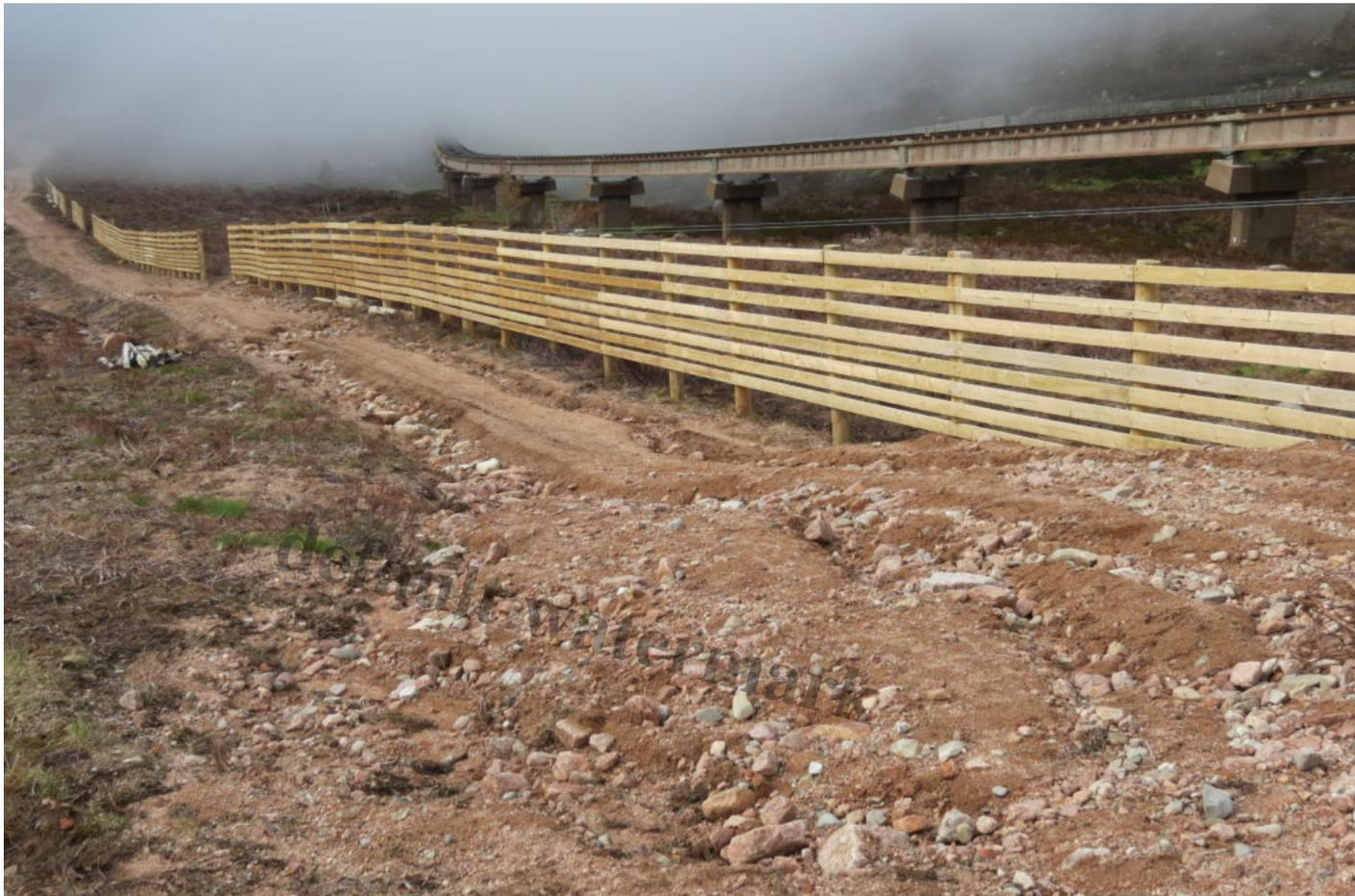
Erosion, including gullying at the top of the new bulldozed track
