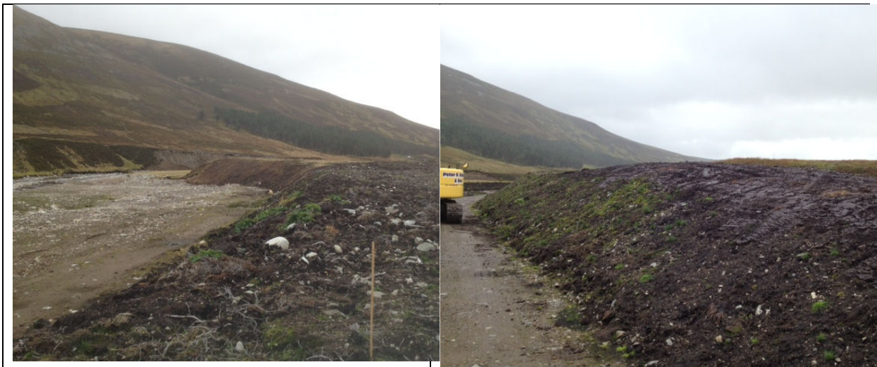
Picture 1 eyebrows removed from terrace to the south west of intake. The lower area in the picture will undergo secondary planting.
