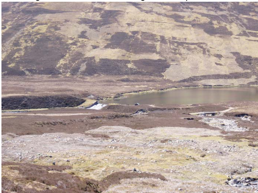
Figure. 6- Existing dam/weir (to be enlarged) and intake area.
