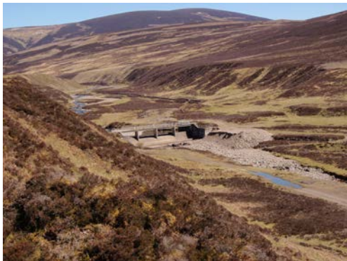
Fig. 4- Existing SSE Dam
