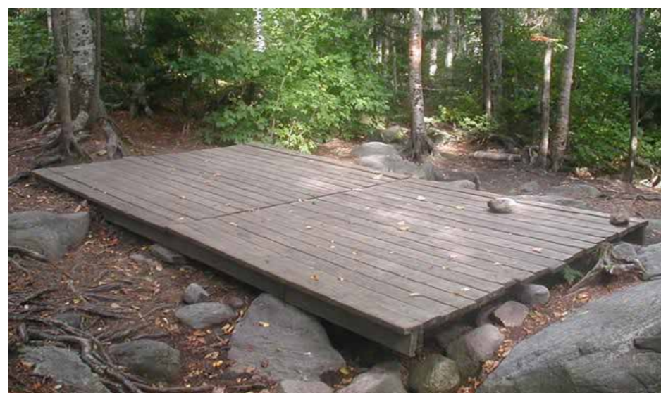
Camping Platforms - approx. size 3m x 3m, placed in pitches which are in steep or damp areas to allow tents to be pitched
