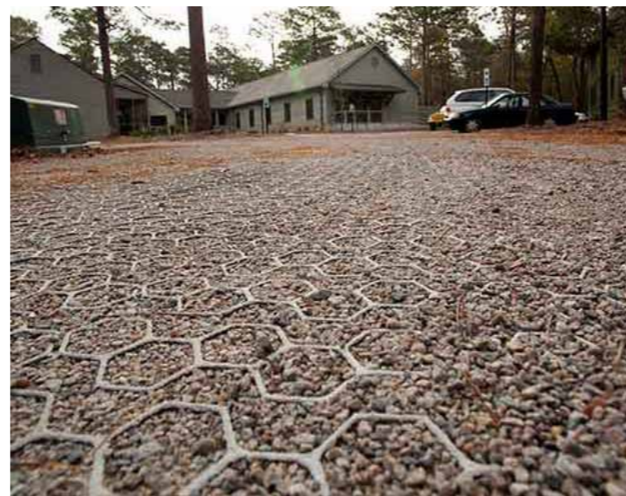
Car Park Area Surfacing will be a plastic paving grid infilled with gravel and a raised timber kerb detail around the edge.
