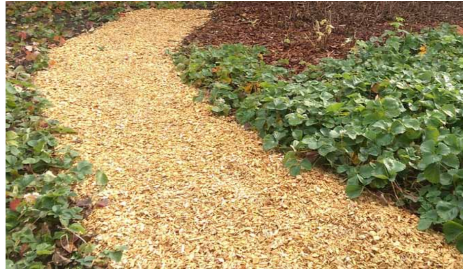
Secondary footpaths leading to camping pitch areas from the main footpaths will be surfaced with bark, and a natural edge to meet adjacent vegetation.
