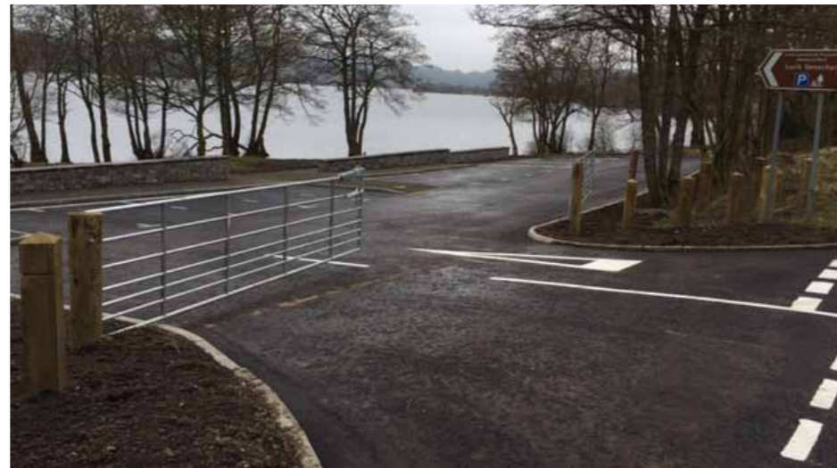
Vehicle Barrier - to control vehicle access into the site. Barrier will be a galvanised steel, agricultural style gate.
