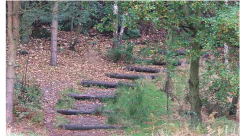
Steps to access higher areas will be constructed of heavy timber units / railway sleepers, held in place with half round timber stakes, treads to be well-rammed soil, surfaced with compacted hardcore.
