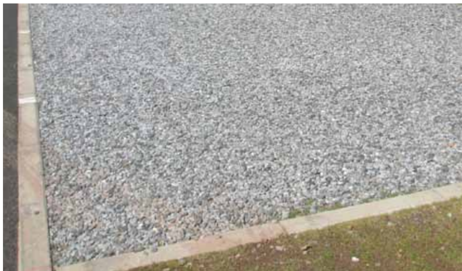
Access Road Surfacing will be compacted hardcore gravel similar to the existing surface, with a natural edge finish to meet the adjacent grass. The edge between the access road and the parking spaces will be delineated with a flush concrete kerb.
