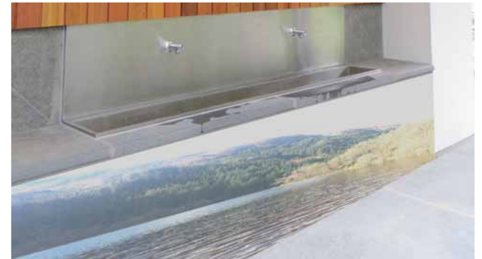
Washing Up Area - Sink and Standpipe - approx. 1.2m long wash trough unit, front, back and sides clad with aluminium 'dibond' panels which are printed with woodland or loch-side images to reflect the setting. One tap at either end of sink unit. One standpipe tap to be located on the end face of unit to allow water receptacle to be placed on ground while filling up.
